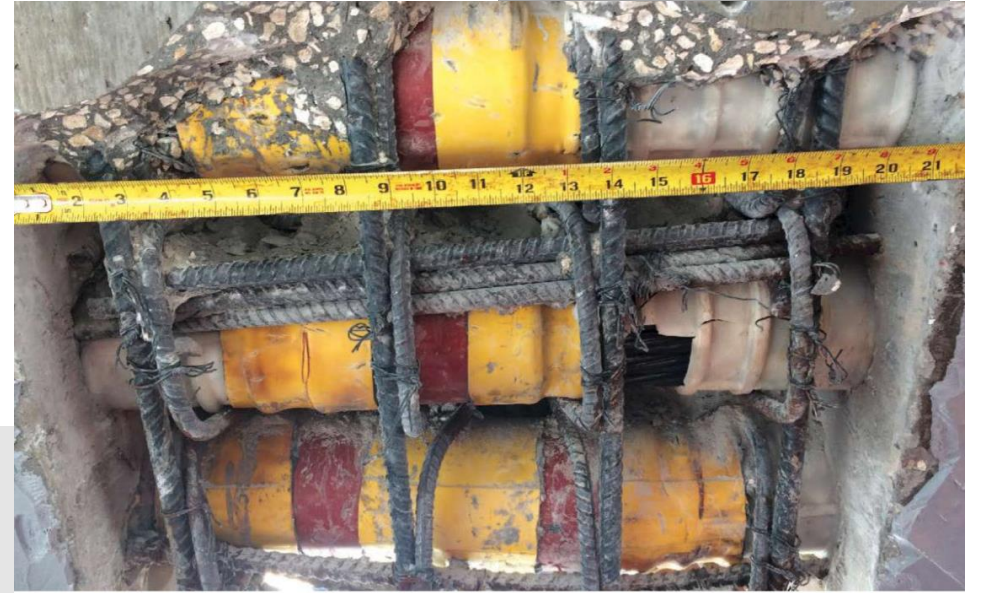
Ultra-high-performance concrete was used for the repair of a midspan spliced U-girder closure pour. Photo: SEMA Construction
