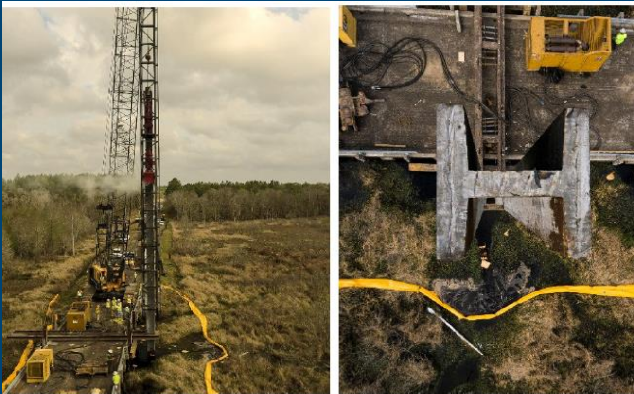
Pile driving photos courtesy of Cor-Tuf UHPC
