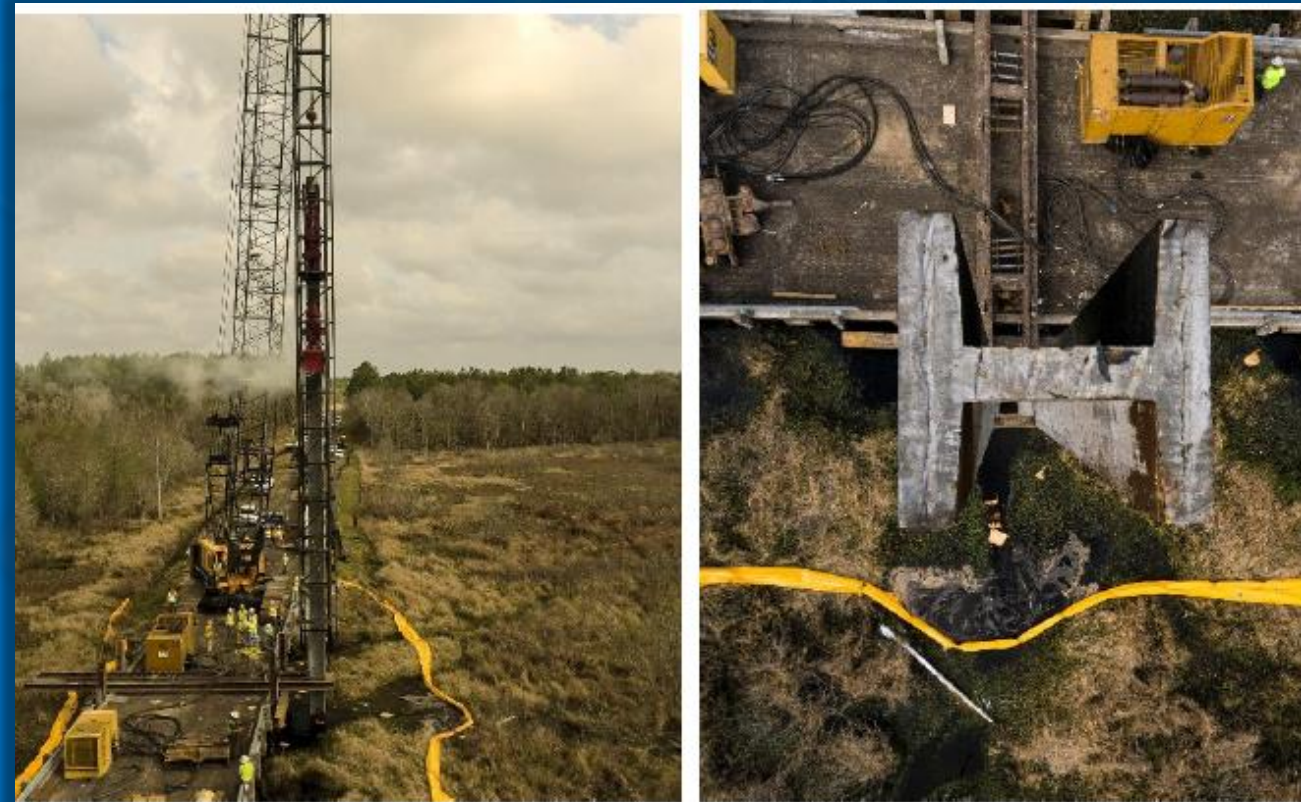
Pile driving photos courtesy of Cor-Tuf UHPC
