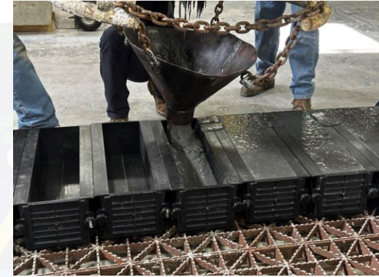
Casting of UHPC mixture from one end
