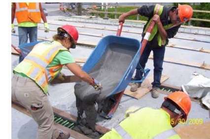
Different casting methods in UHPC construction (Source: Cor-Tuf, New York DOT)
