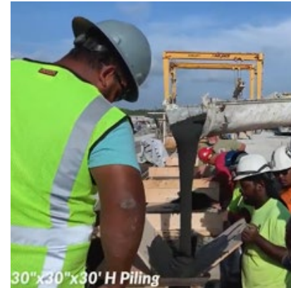
Casting of H-piles in H-direction (photo courtesy: Cor-Tuf)
