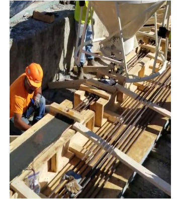
Casting H-piles in I-direction (photo courtesy: Smart UP)
