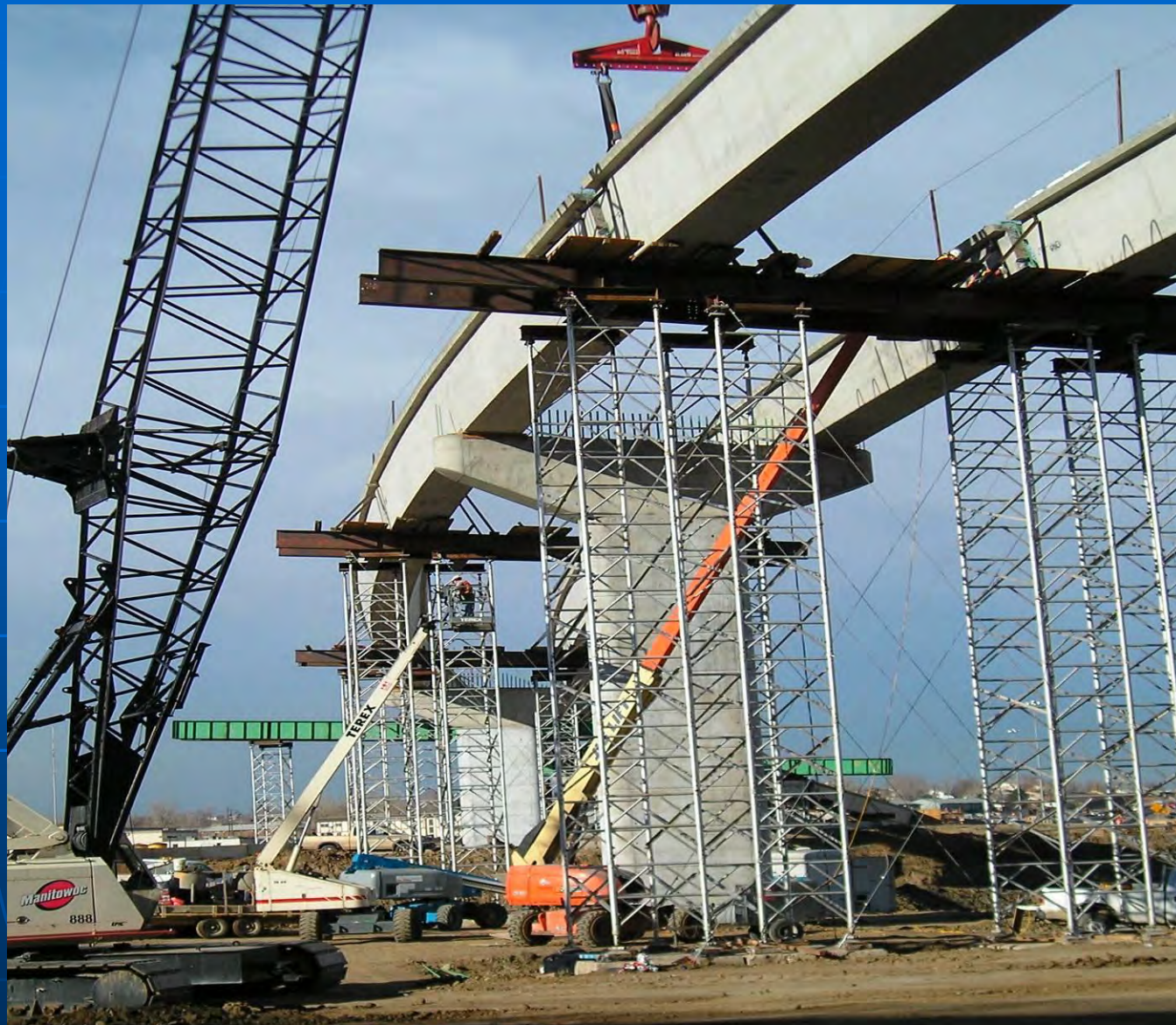
Ramp K on 45' Falsework Towers @ Pier 5
