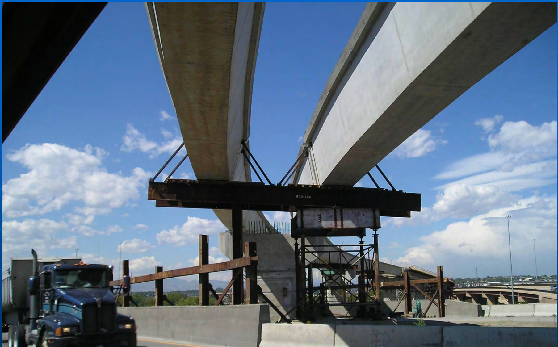
Ramp Y Safety Rail protecting Falsework Bents Adjacent to IH76 Traffic
