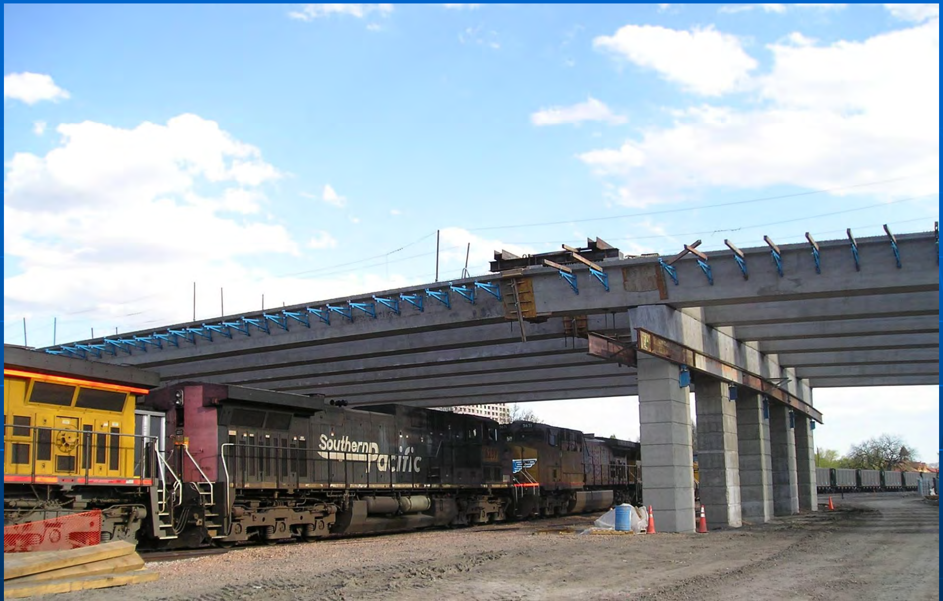
Bijou Street Bridge Span 3 set over Rail Yard, 148' Clear Opening
