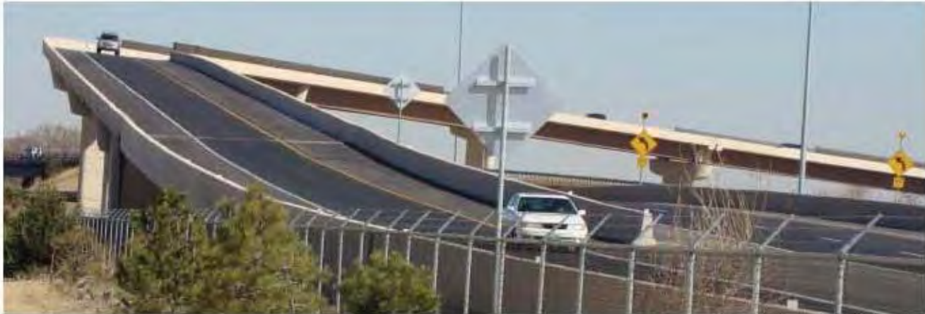
Photo courtesy of Summit Engineering Group Inc.
