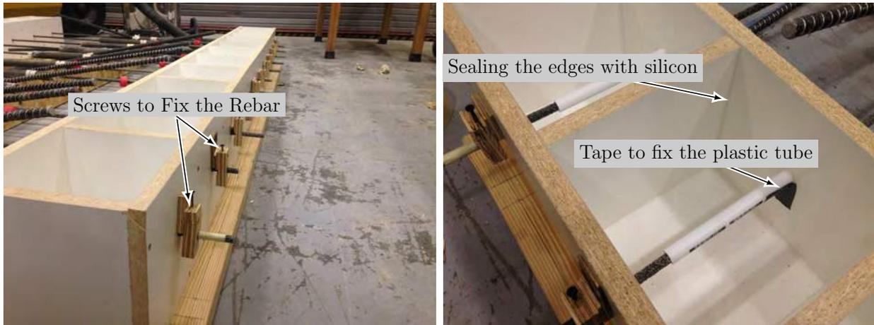
Figure 4.18: Fixing the rebar and the plastic tube
