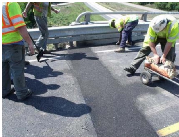
Fig. 10: Asphalt Plug Joints
