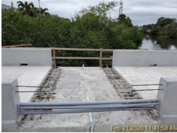
Figure 2.4: Link-slab photos prior to setting reinforcement
