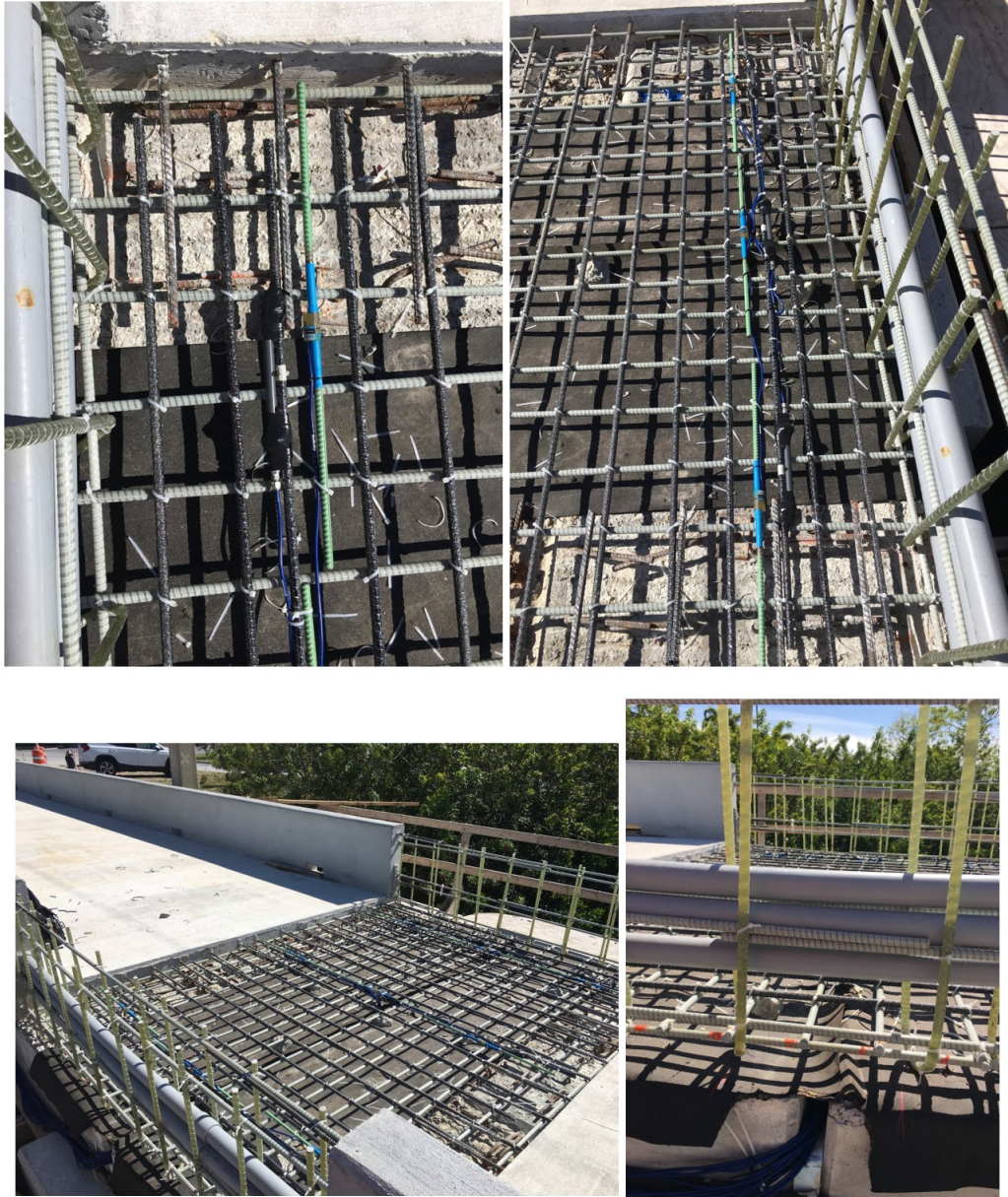
Figure 2.3: Link slab reinforcement and embedded sensors
