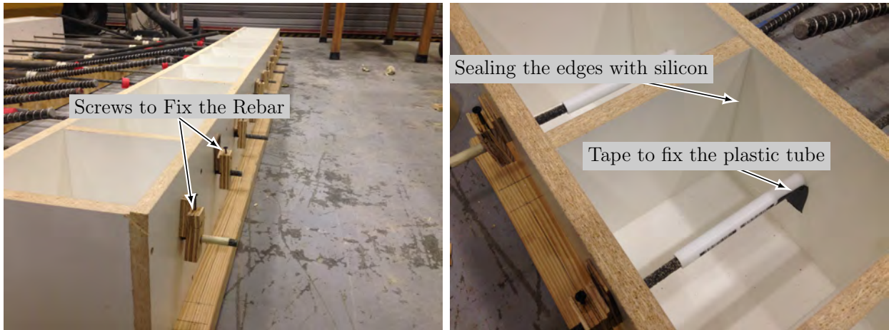
Figure 4.18: Fixing the rebar and the plastic tube
