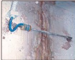
• Model 4420 Crackmeter installation.
