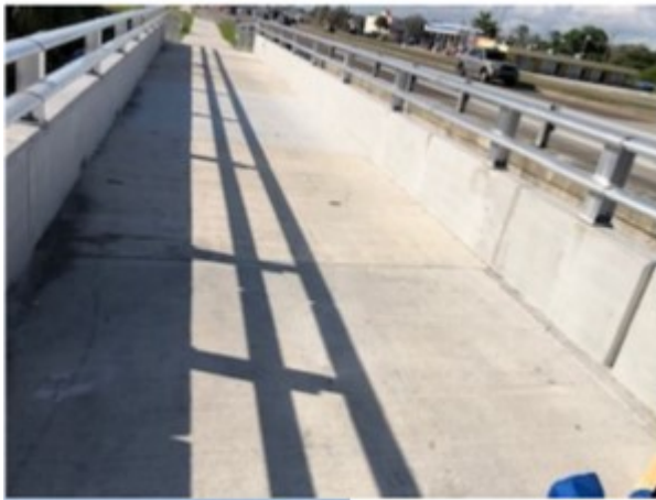
Figure 2.5: Finished link slab and close up view
