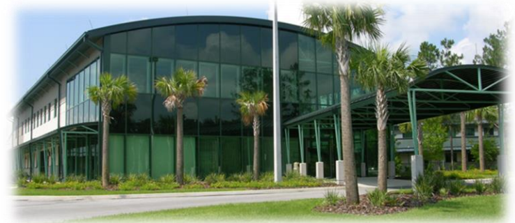
State Materials Office
