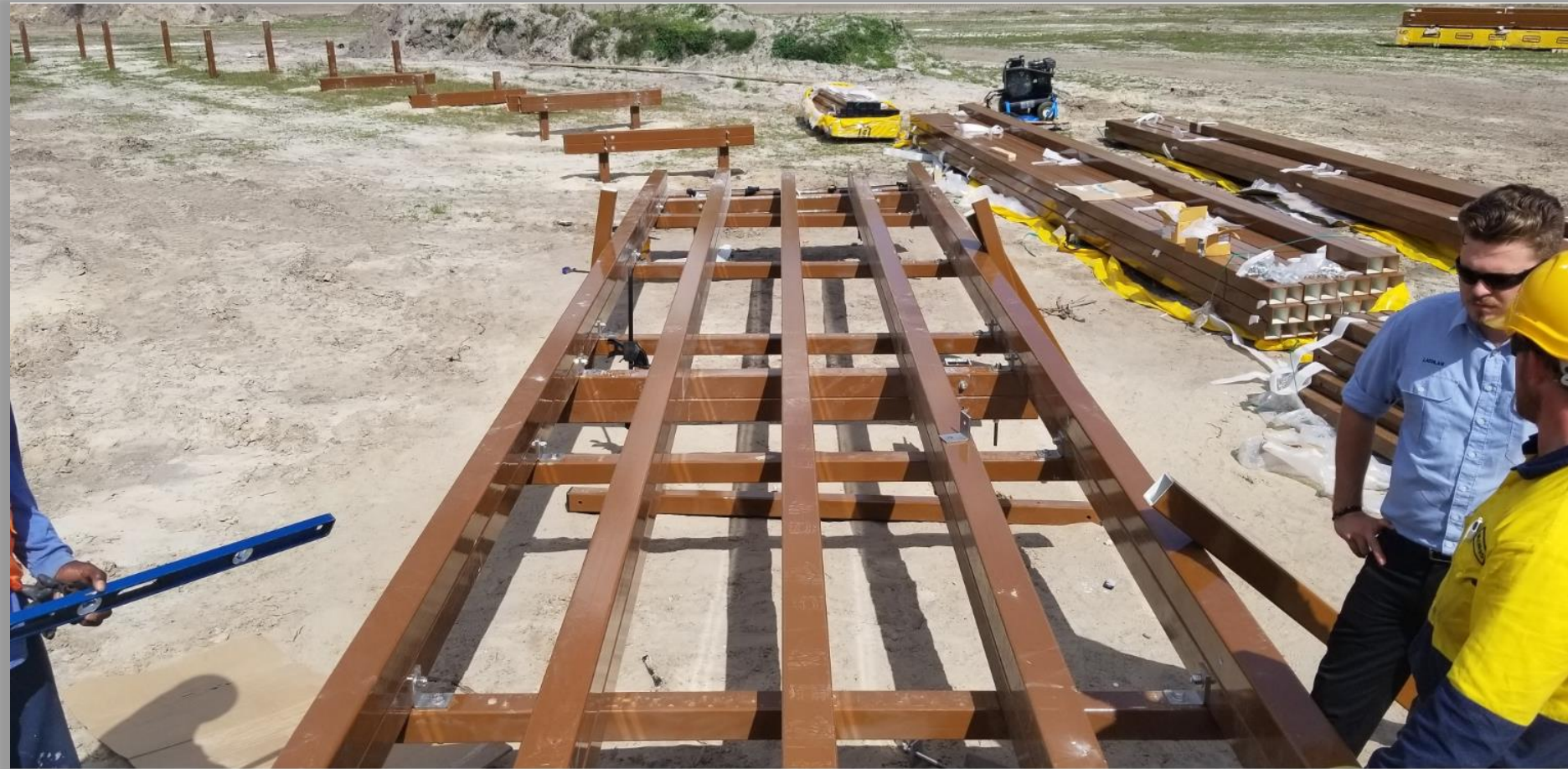
Installing the Bonded Bearers and Stringer Sections
