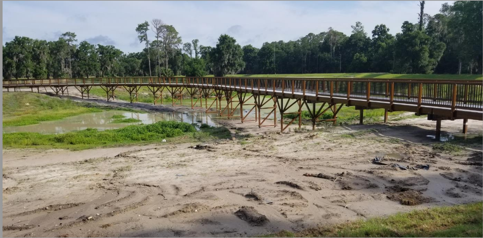
A completed pond walk-over. Waiting to flood the cell
