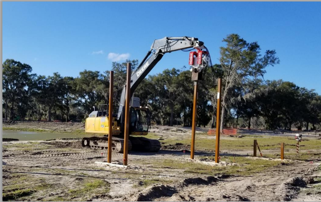
Pile Driving 5"x 5" Composite Sections
