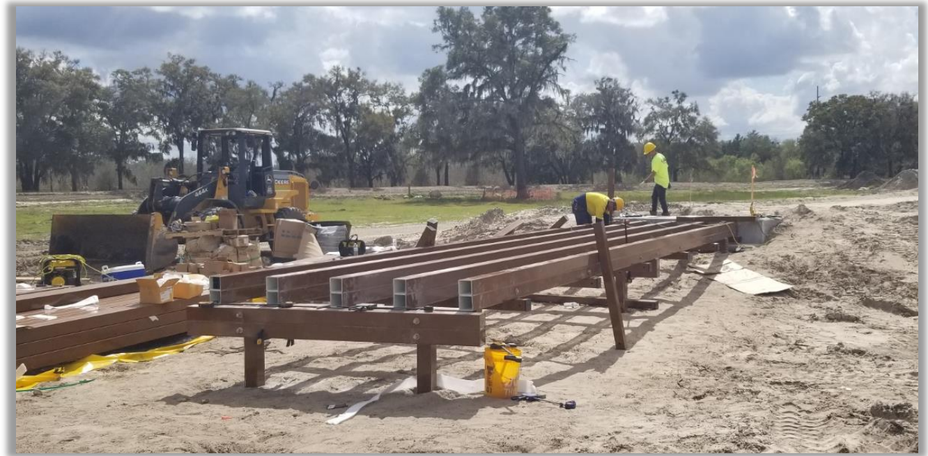
Installing the Bonded Stringer Sections
