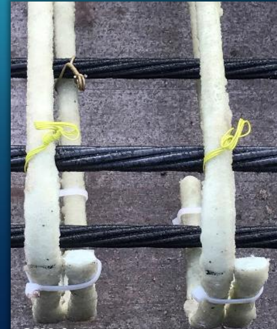
GFRP Stirrups ties to CFRP strands (2016)
