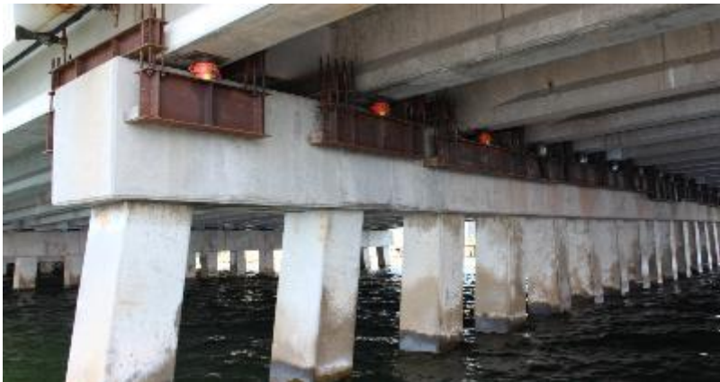
CFRP Girder Bearing Repair
