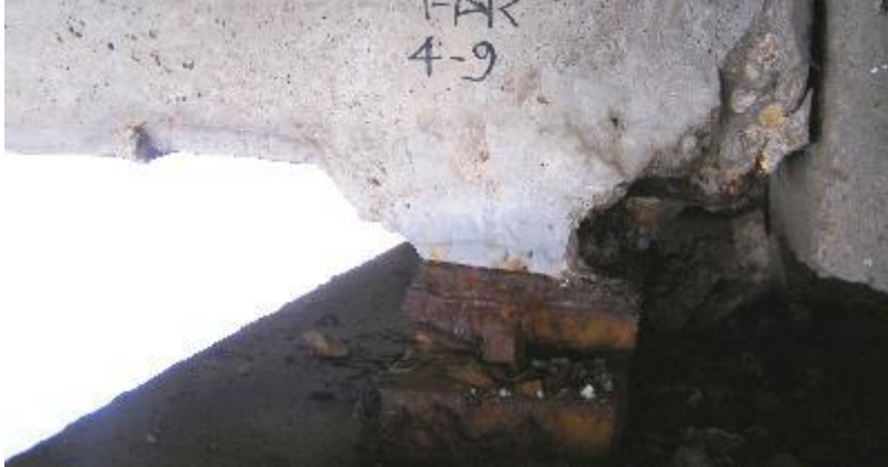
CFRP Girder Bearing Repair
