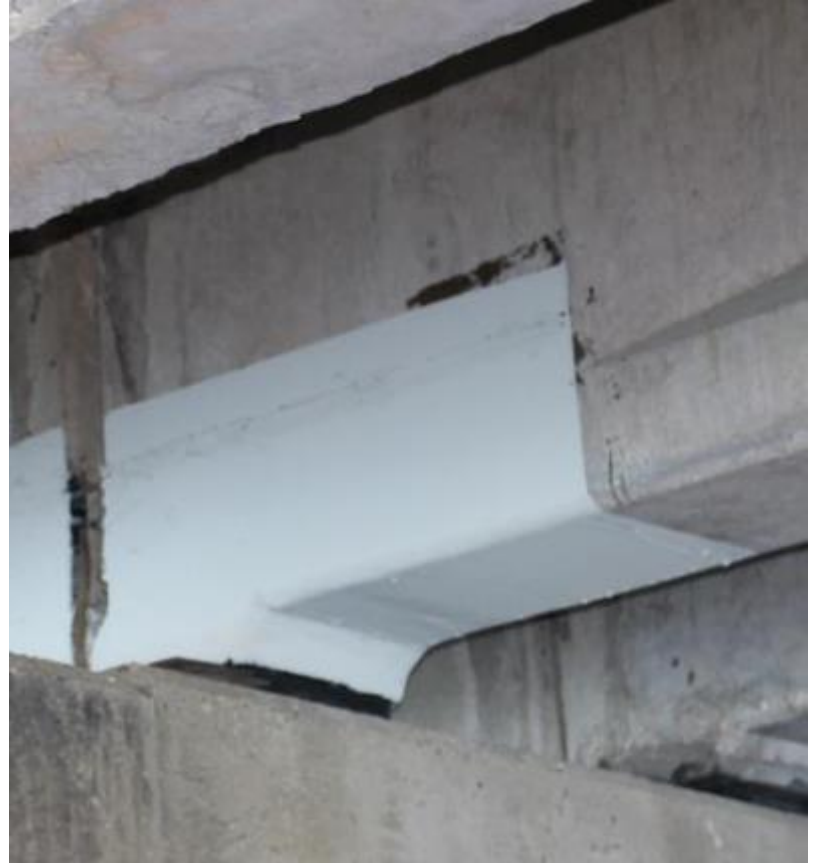
CFRP Girder Bearing Repair
