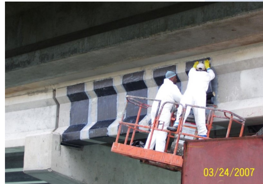
Strengthening – Corrosion Damage
