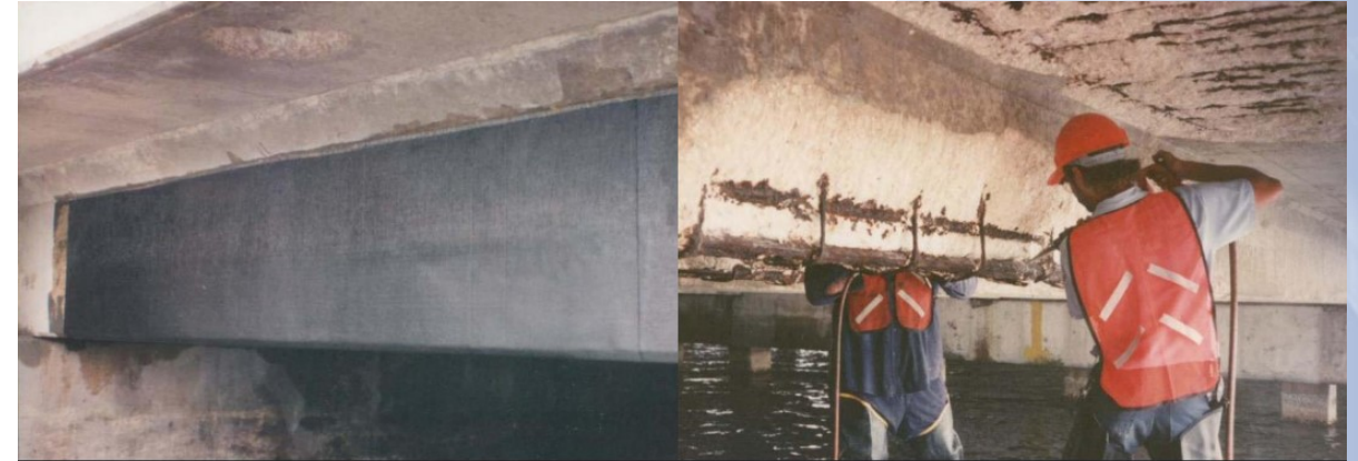
Strengthening – Corrosion Damage
