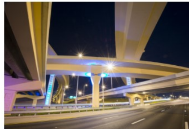
Image courtesy of BCC Engineering
