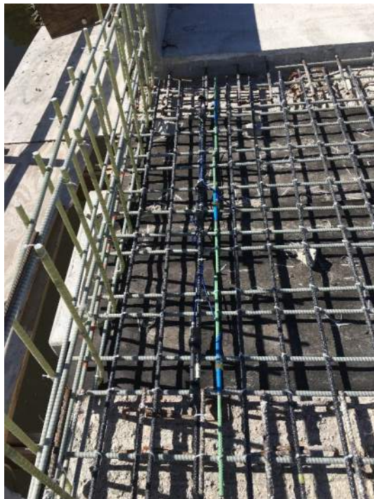
Photo 8 & 9: Typical Vibrating Wire Strain Gauge Sensor on BFRP rebar with parallel coated steel Sister-Bar (green) at three locations, SE side (left) and mid/centerline (right).
