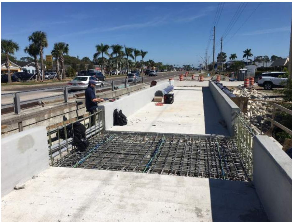
Photo 2: Link-Slab BFRP longitudinal rebar and strain gauges installed 3/6/2020.
