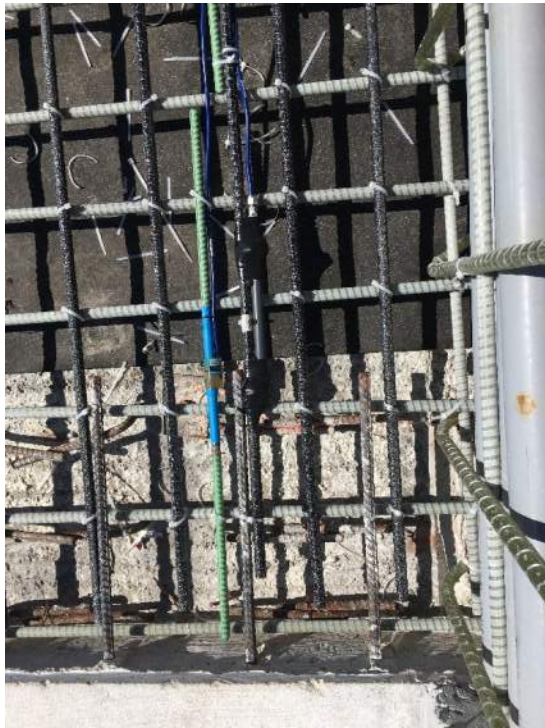
Photo 6 & 7: Typical Vibrating Wire Strain Gauge Sensor on BFRP rebar with parallel coated steel Sister-Bar (green), SE side.
