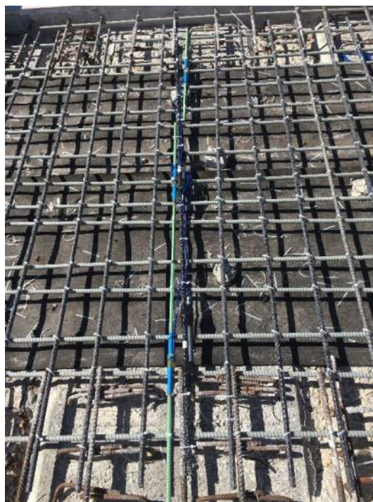
Photo 8 & 9: Typical Vibrating Wire Strain Gauge Sensor on BFRP rebar with parallel coated steel Sister-Bar (green) at three locations, SE side (left) and mid/centerline (right).
