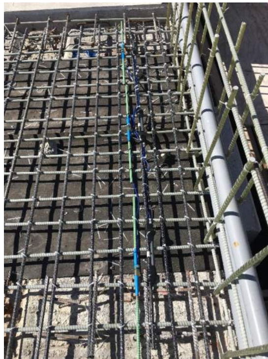
Photo 6 & 7: Typical Vibrating Wire Strain Gauge Sensor on BFRP rebar with parallel coated steel Sister-Bar (green), SE side.
