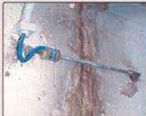
• Model 4420 Crackmeter installation.
