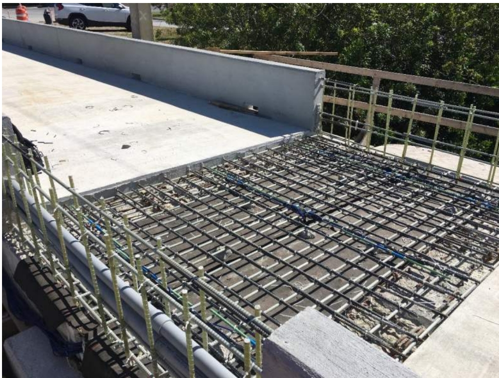
Photo 5: Link-Slab BFRP longitudinal rebar and strain gauges installed 3/7/2020.
