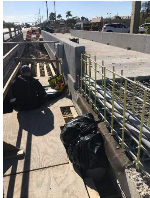
Photo 10 & 11: Installing and setting up data loggers and cable connections
