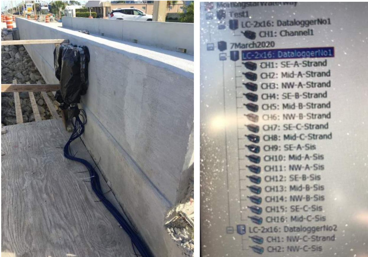
Photo 13: Temporary cable routing to Geokon 8002 Data Loggers ready for link-slab casting scheduled for 3/11/2020
