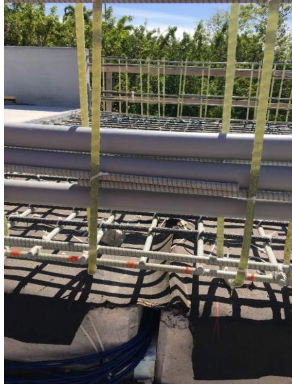
Photo 3 & 4: Link-Slab BFRP longitudinal rebar strain gauge cable routing thru between CIP diaphragms 3/7/2020.
