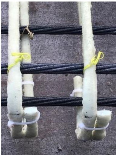
Figure 11: Epoxy and plastic-coated ties
