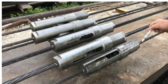
Figure 10: CFCC-Steel coupler installation
