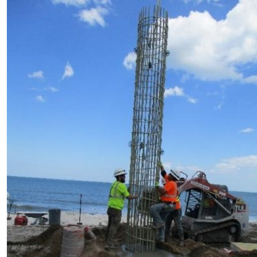
GFRP Secant-Pile Shaft cages for A1A-Flagler Beach seawall (2019)
