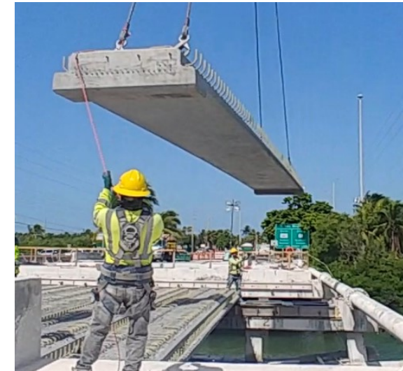
FRP-PC FSB's US-1/Cow Key span replacements (2020)
