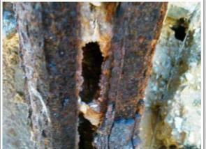
Figure 3 - Corrosion at the joint between two sheet piles showing complete section loss.
