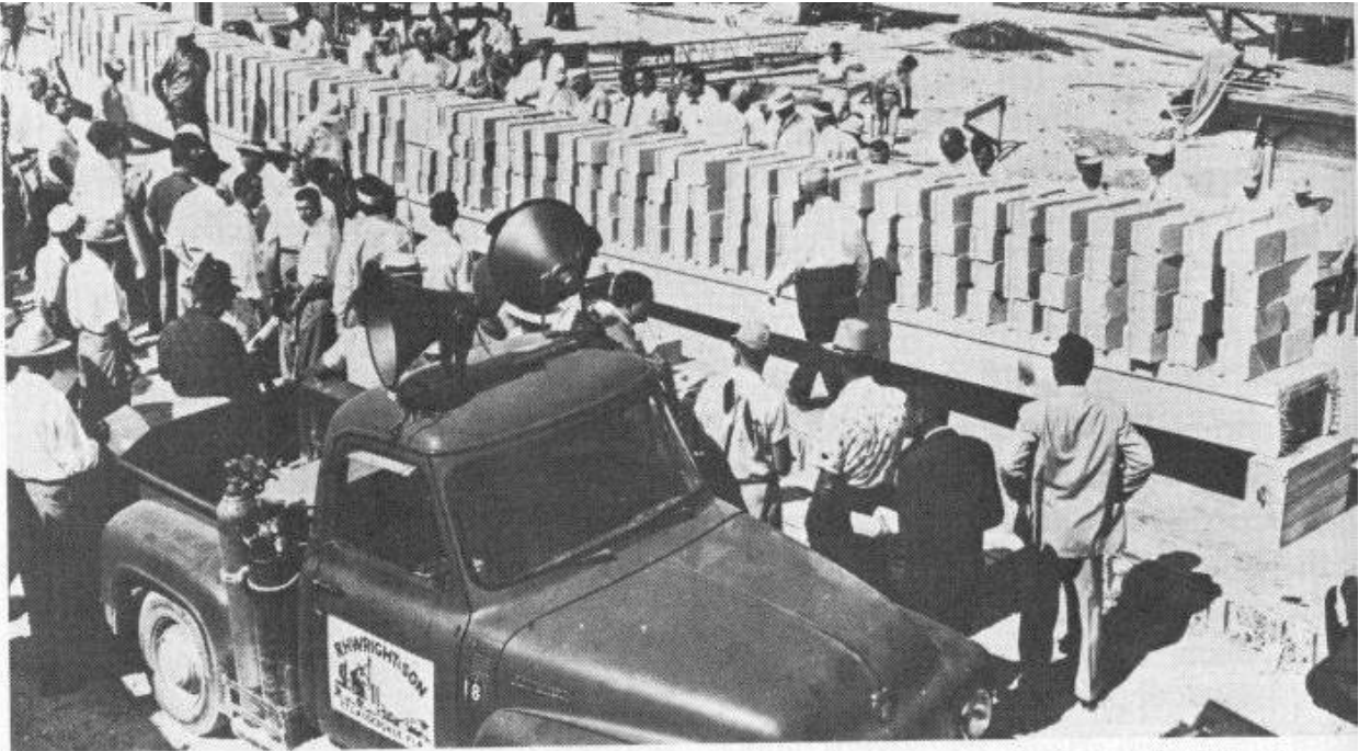
Fig. 25. Demonstration test of 100-ft (30.5 m) long prestressed channel slab at R. H. Wright & Son, Fort Lauderdale, Florida.
