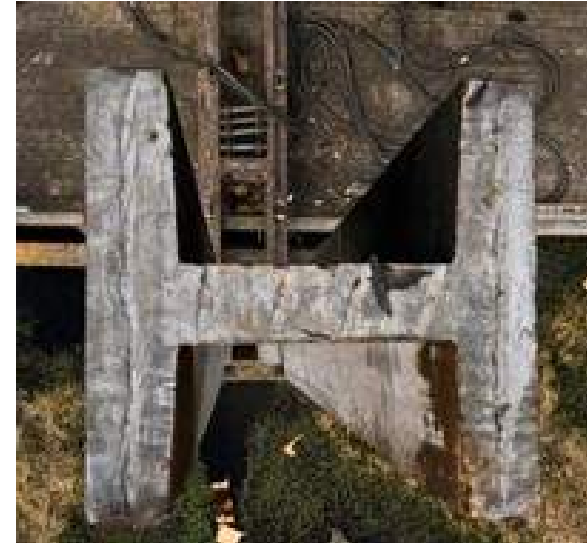
UHPC-PC H-Pile for CR-339 demonstration (2020)
