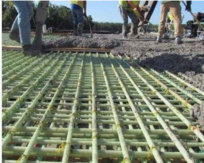
GFRP rebar for deck & substructure of Halls River Bridge (2017-19)
