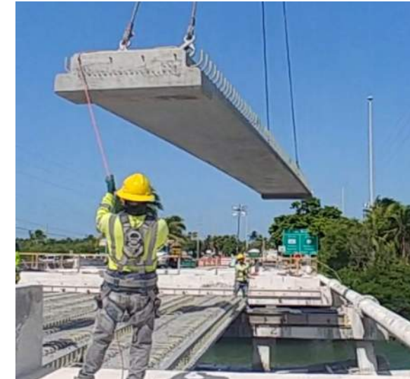
CFRP-PC FSB's US-1/Cow Key span replacements (2020)
