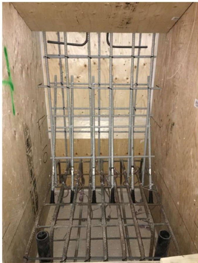
Figure 4.14: Typical GFRP wall mesh at exterior location
