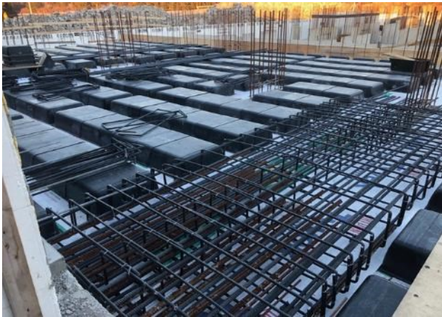
GFRP -RC Waffle flooring slabs
