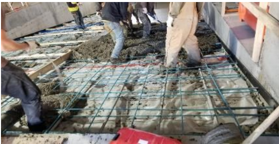
GFRP-RC Slab-on grade
