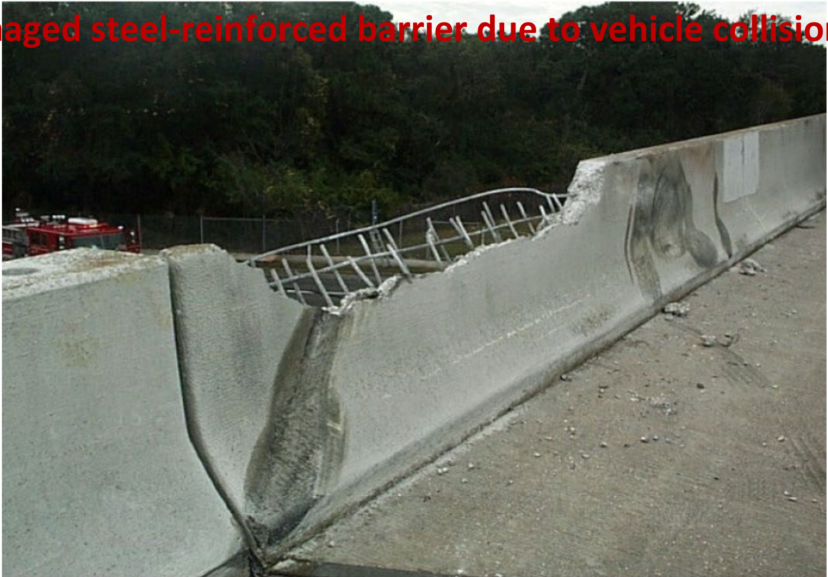
Florida Bridge Railing Failure
