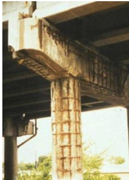
Corrosion Damage to RC Columns
