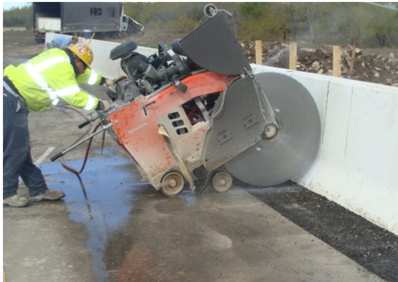
Saw-cut the defected segment
