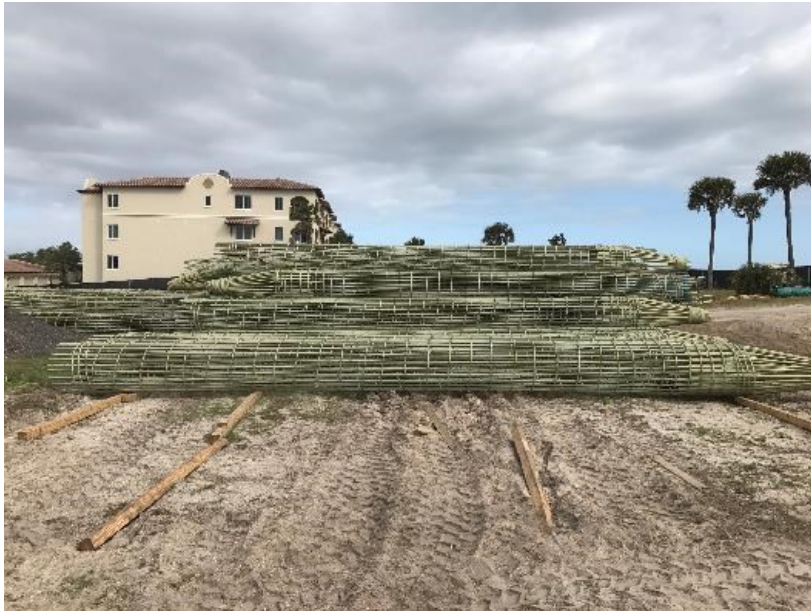
Cages of 25 mm GFRP bars and 15 mm GFRP Spirals
