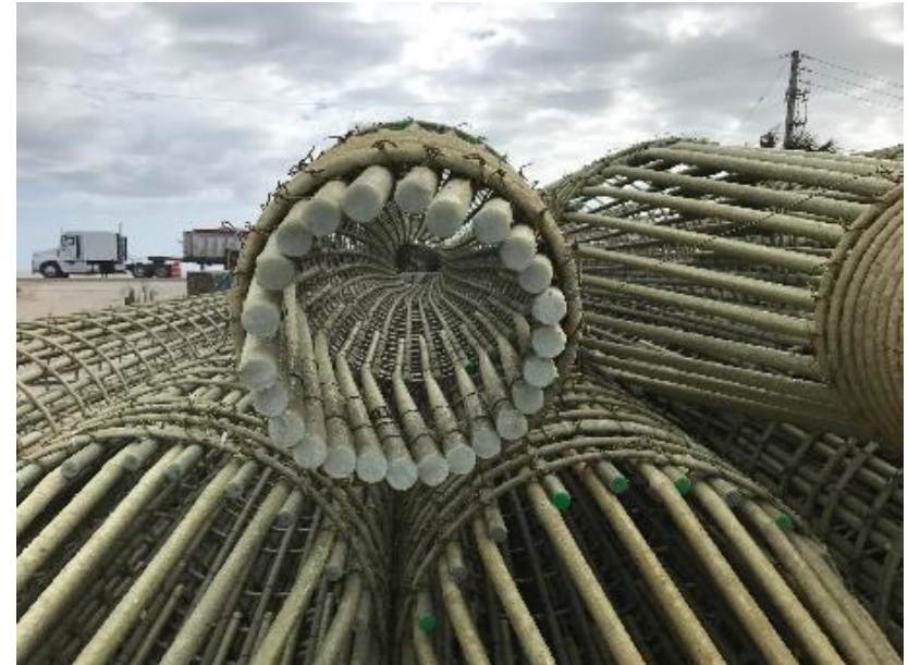
Cages of 25 mm GFRP bars and 15 mm GFRP Spirals
