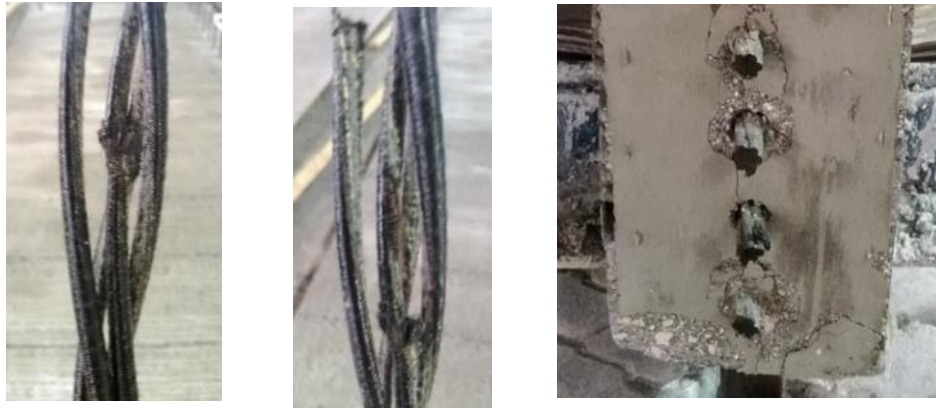
(a) & (b) CFRP strand failed during tensioning; (c) cracking following strands release.
