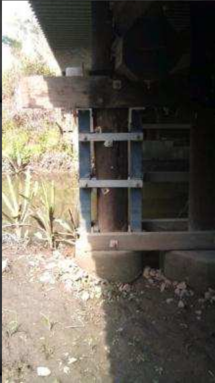
Pile Strengthening
