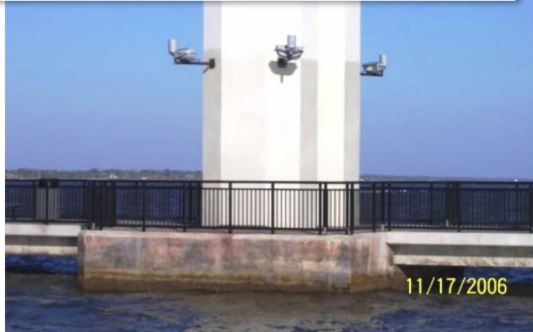
Figure 3: View of Pier 12 showing footer and two octagonal columns of Bridge 890145. Stainless steel 2101LDX used on footer and column.
