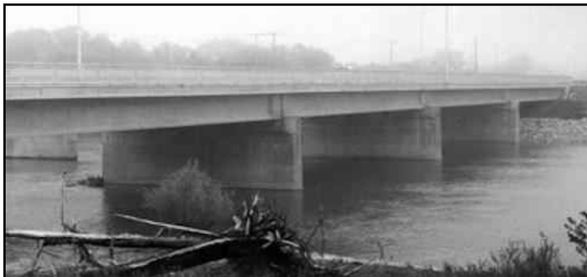
Figure 2.30: Taylor Bridge, Manitoba, Canada (ISIS Canada, 2009)
