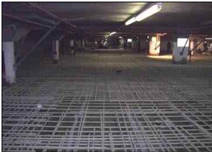
Figure 2.36: La Chancelière Parking Garage
