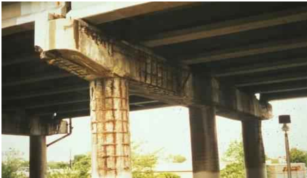
Figure 2.7: Concrete structure deteriorated by the corrosion of steel reinforcement
