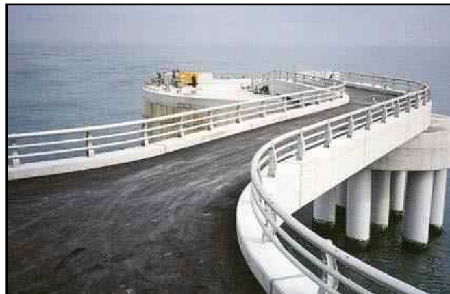
Figure 2.25: Haranomachi thermal power plant outfall Bridge
