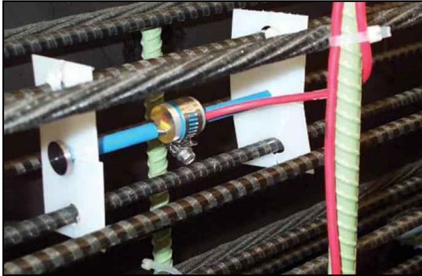
a) Leadline tendons and CFRP strands in reinforcement cage of double-T girders
