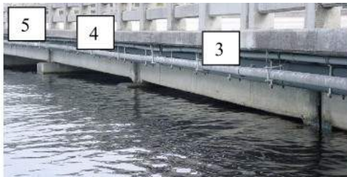
Report: BDV31 977-01 (University Blvd Bridge, 2011)
