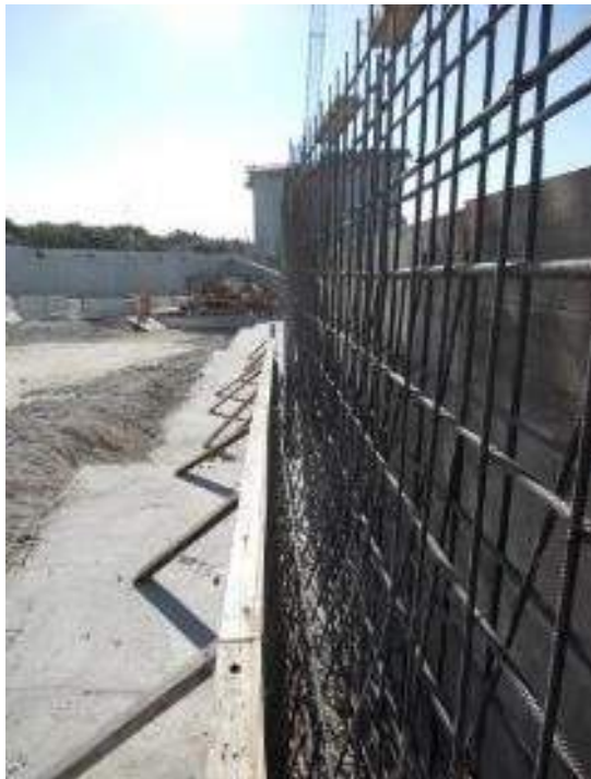
Wall 6 under construction & Typical Cross-section using Basalt FRP rebar
