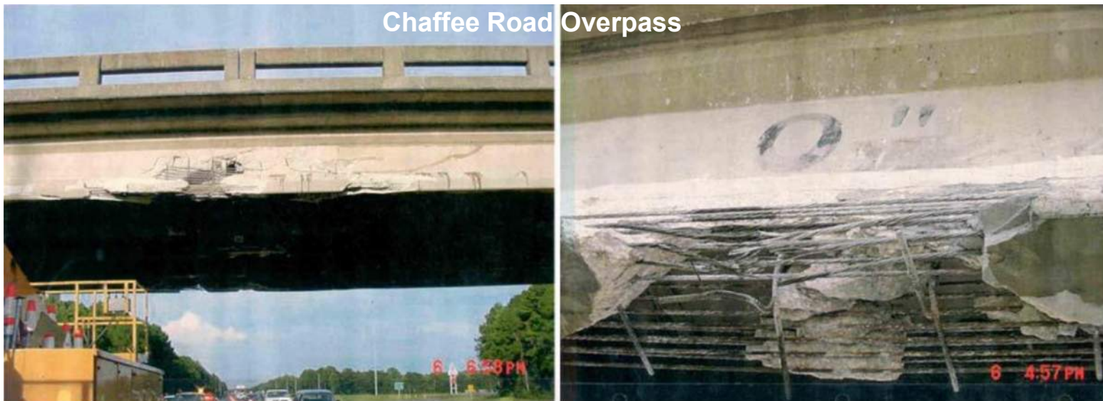
BDV31 977-01: Figure 227—Girder damage from vehicle impact in July of 2001
