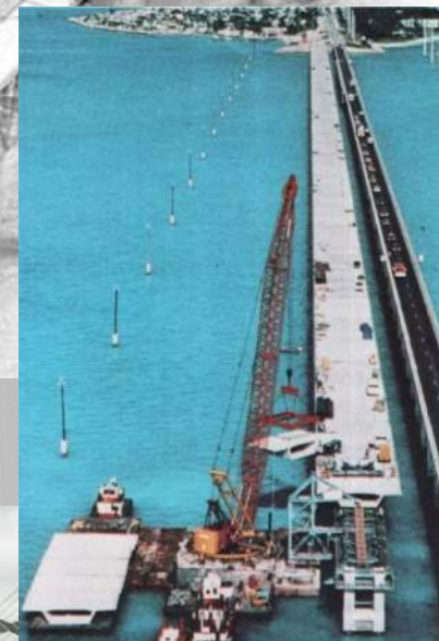
Fig. 1. Long Key Bridge — A precast segmental, post-tensioned, span-by-span structure. (Courtesy of Figg and Muller Engineers Inc., Designer)
