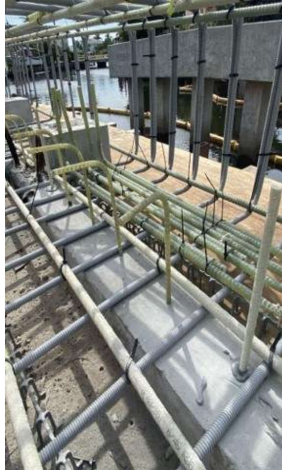
IBIS-Waterway Bridge GFRP placement at End-Bents atop Precast Seawall-Panels, and at Intermediate-Bents
