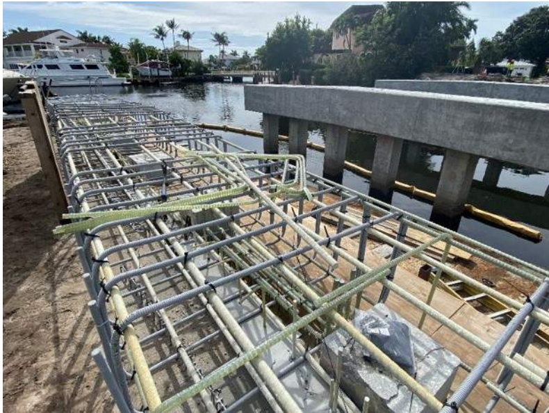
IBIS-Waterway Bridge GFRP placement at End-Bents atop Precast Seawall-Panels, and at Intermediate-Bents
