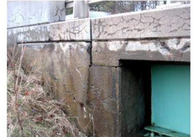
Map cracking.
