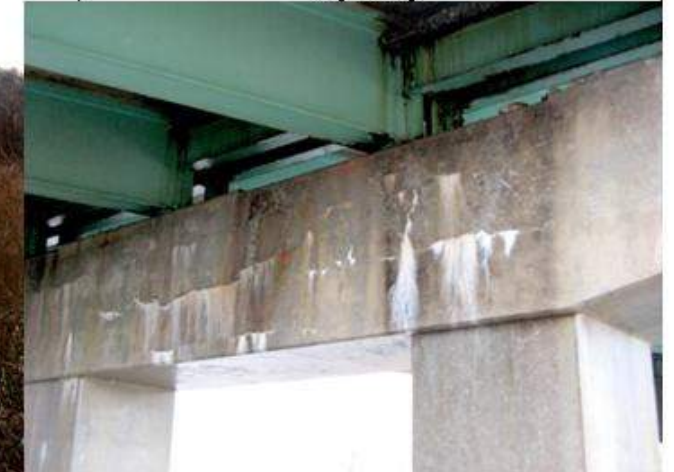
SW'ly face of SW'ly pier.
