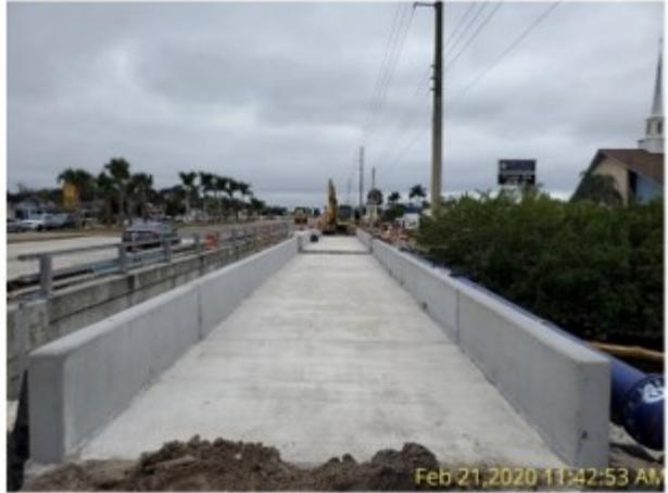
Figure 2.4: Link-slab photos prior to setting reinforcement
