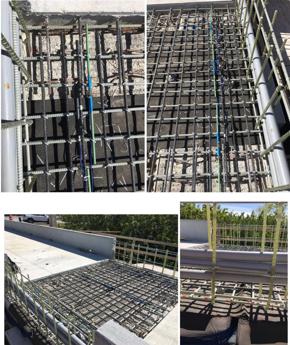
Figure 2.3: Link slab reinforcement and embedded sensors
