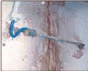
• Model 4420 Crackmeter installation.
