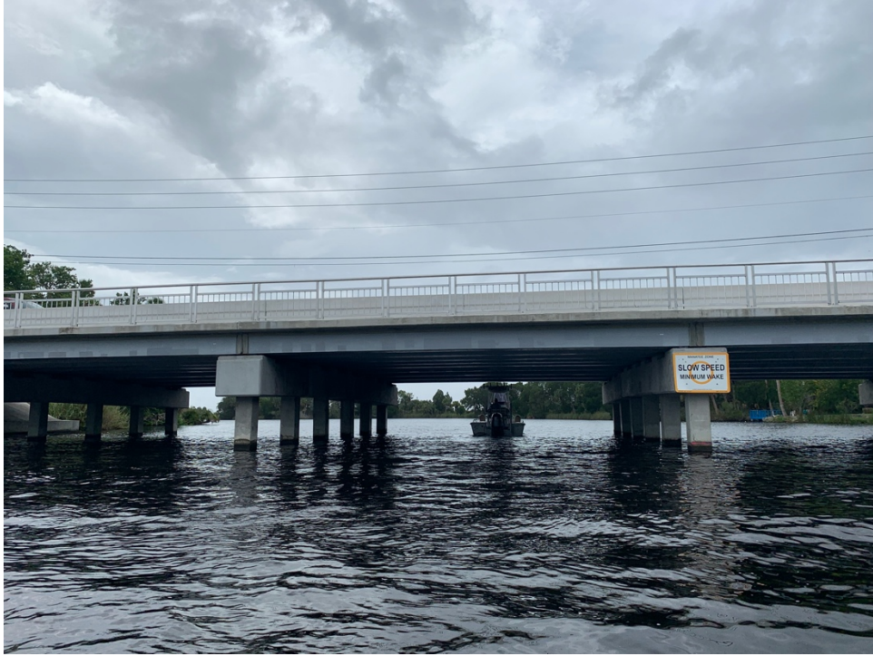
Figure 2: Span 3, looking north
