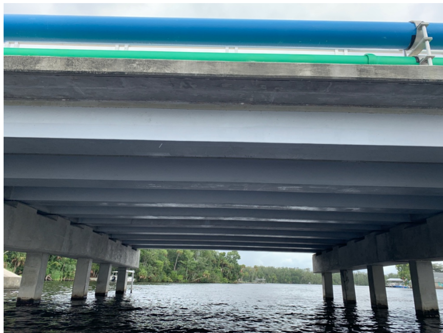
Figure 12: Span 4, looking south
