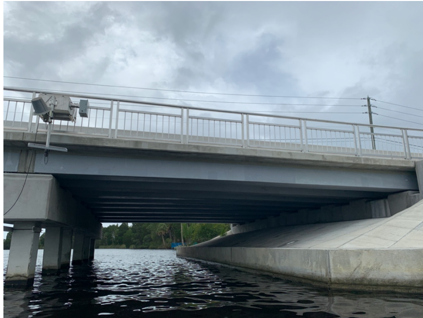
Figure 11: Span 5, looking north
