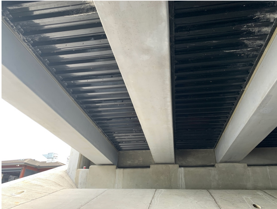
Figure 9: End Bent 1, looking west
