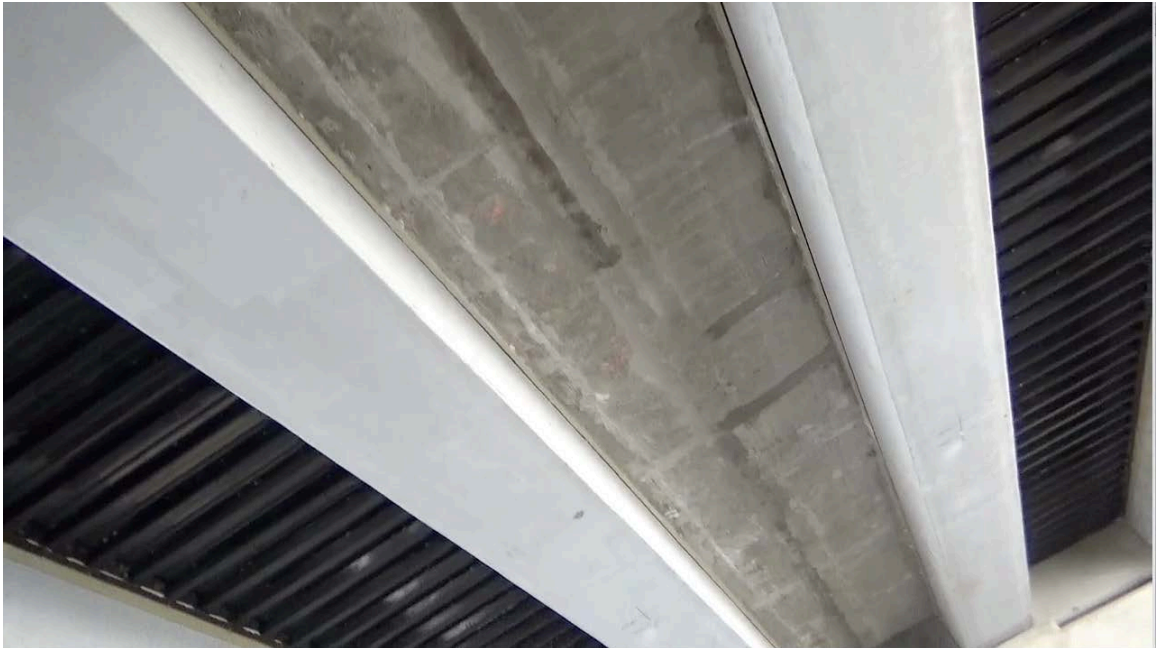
Figure 35: Bottom of slab at construction joint, looking east; (a) Span 4, at three months, (b) Span 5, at two years
