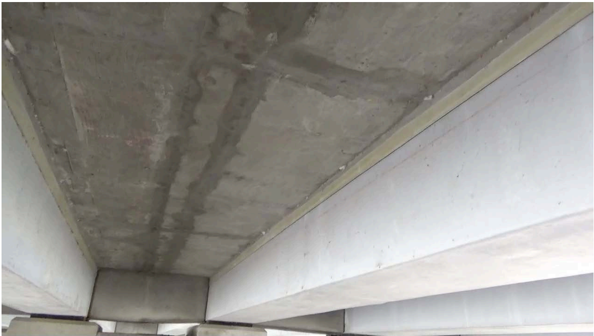
Figure 34: Bottom of slab at construction joint, Span 1; (a) looking northwest, at nine months, (b) looking east, at two years
