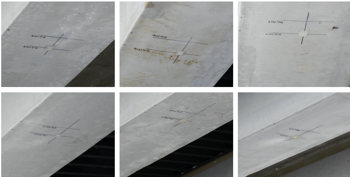
Figure 13: Patches on beams where strain gages were placed for load test
