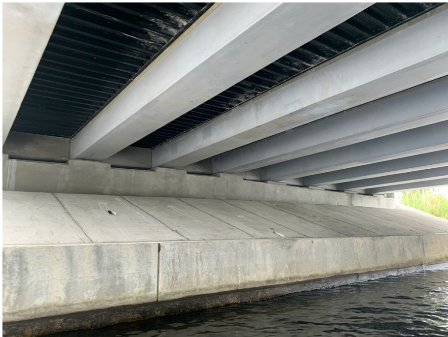
Figure 10: End Bent 1, looking northwest
