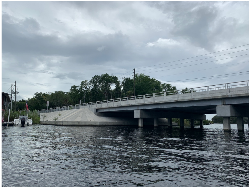
Figure 1: Halls River Bridge, Spans 1 and 2, looking northwest
