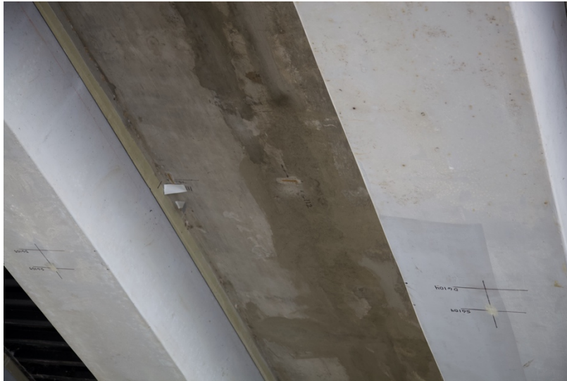
Figure 28: Slab at construction joint in Span 1, near SG112 from load test; (a) at three months, (b) at two years
