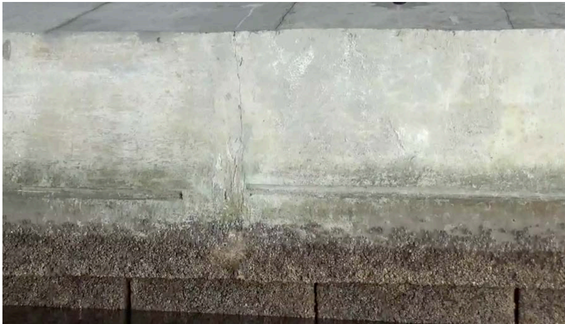
Figure 36: End Bent 6, crack in sheet pile wall cap; (a) at three months, (b) at two years
