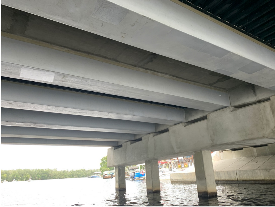
Figure 5: Span 2, looking southwest at Bent 2
