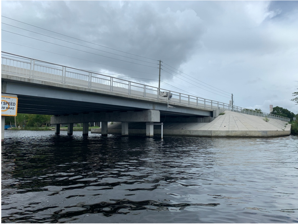
Figure 3: Spans 4 and 5, looking northeast
