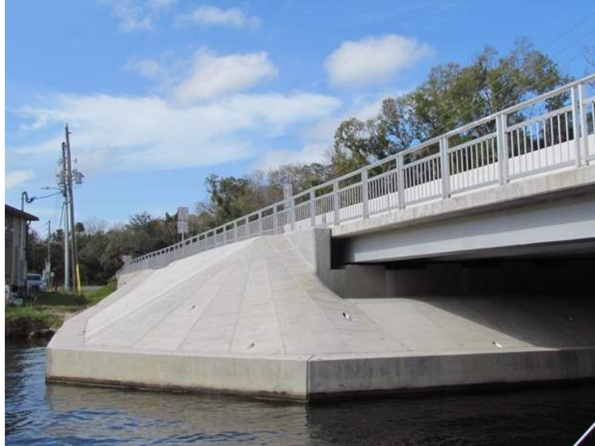
Figure 8: Slope pavement and sheet pile wall
