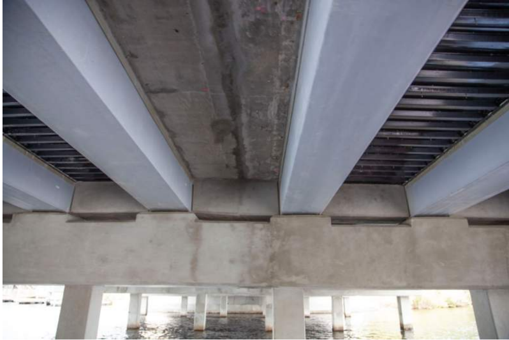
Figure 27: Span 4 underside, looking west at Bent 4
