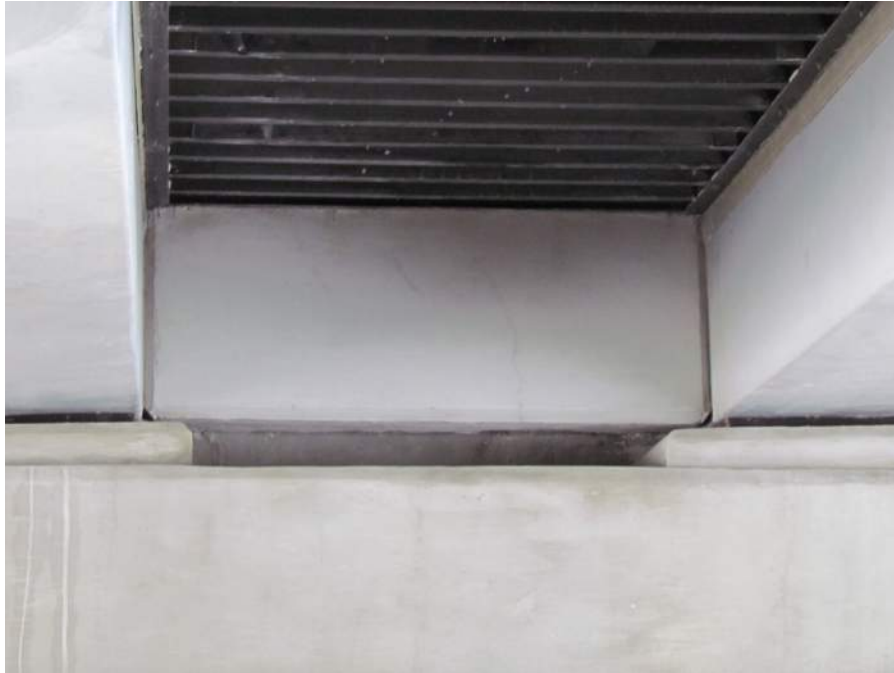
Figure 32: Diaphragm in End Bent 1 at 3 months, looking west
