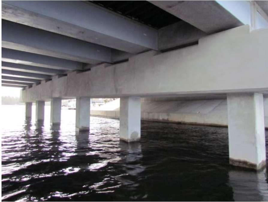
Figure 34: Bent 2 at 3 months, looking southwest
