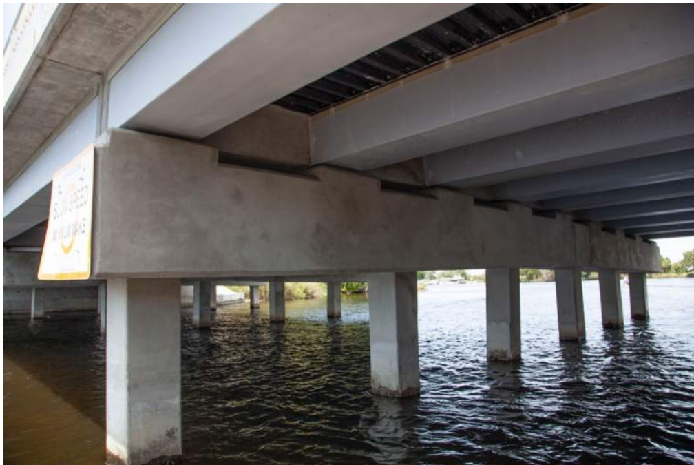
Figure 22: Span 4, looking northwest at Bent 4, view from south side
