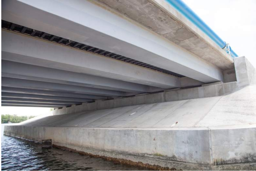
Figure 30: End Bent 1 at 6 months, view from north side, looking southwest
