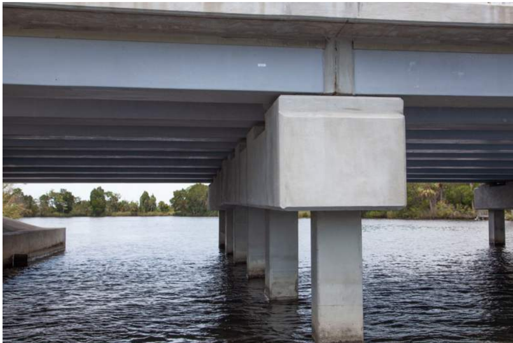
Figure 16: Bent 2, looking north, view from south side
