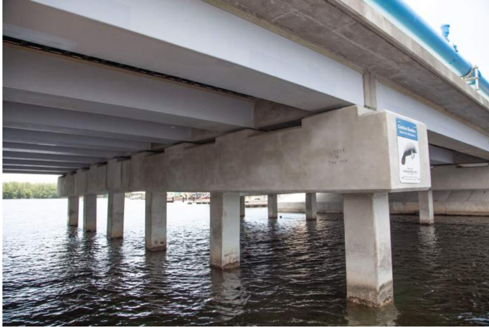
Figure 21: Span 3, looking southwest at Bent 3, view from north side
