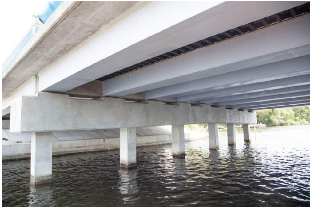
Figure 28: Span 4 underside, looking southeast at Bent 5, view from north side
