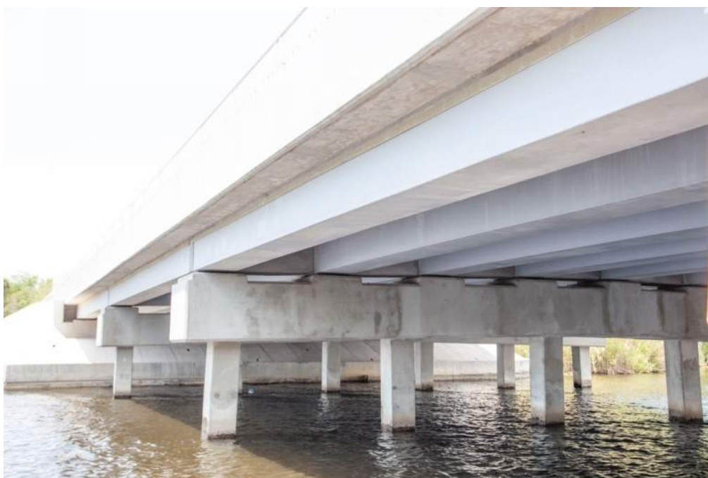
Figure 26: Span 3 underside, looking northwest, view from south side
