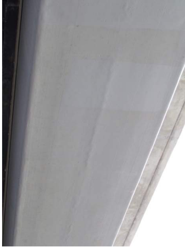
Figure 4: Ripples on underside of HCB
