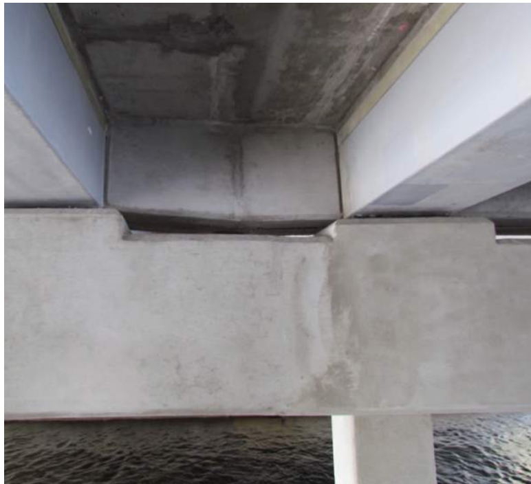
Figure 5: Gel coat patch on HCB
