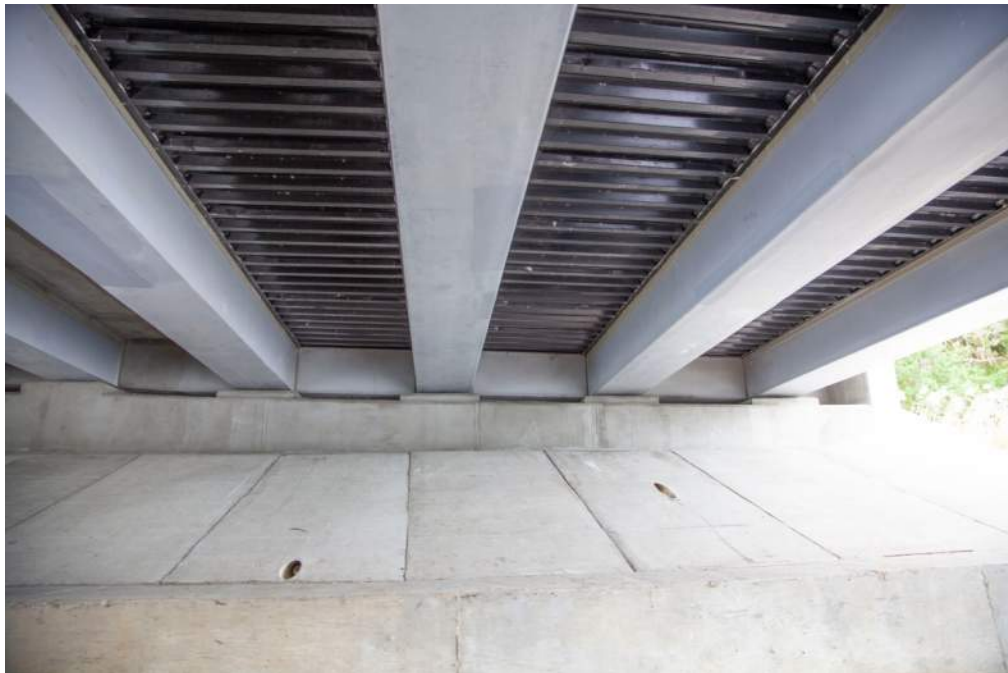
Figure 31: End Bent 1 at 6 months, looking west
