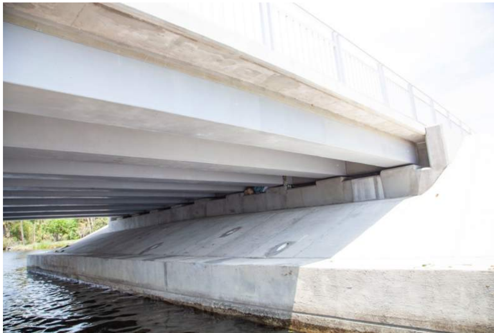
Figure 39: End Bent 6 at 6 months, view from south side, looking northeast
