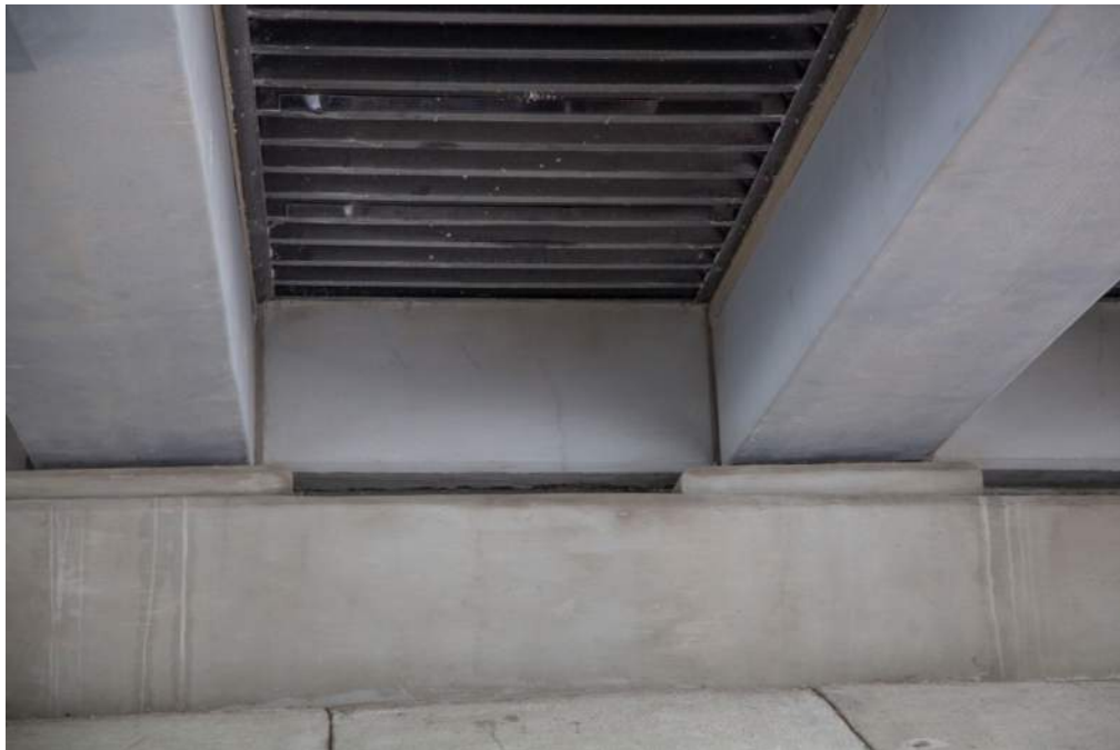
Figure 14: End Bent 1, looking west
