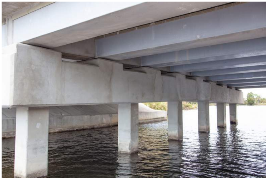
Figure 18: Span 2, looking northwest at Bent 2, view from south side
