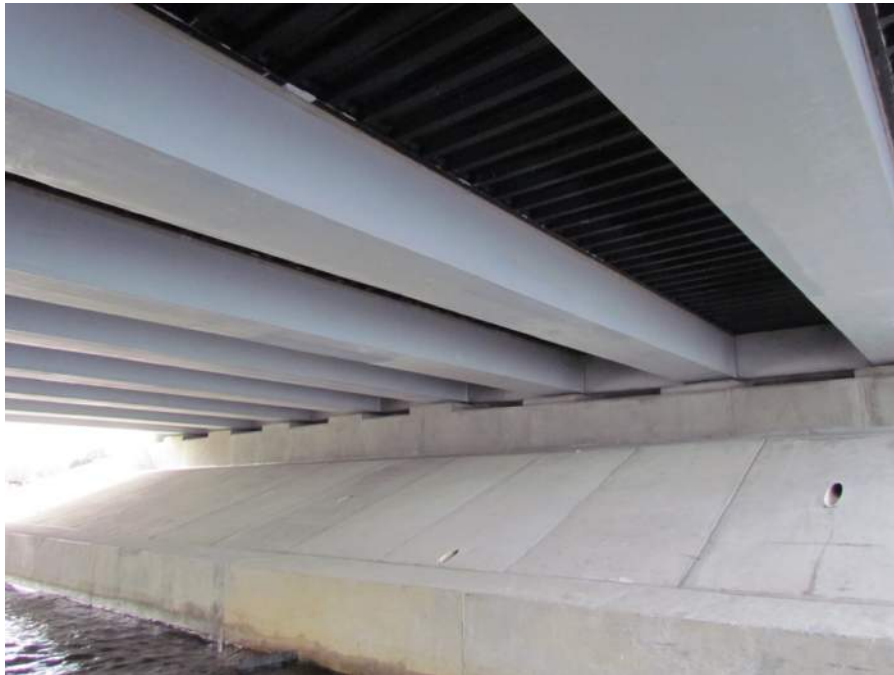
Figure 29: End Bent 1 at 3 months
