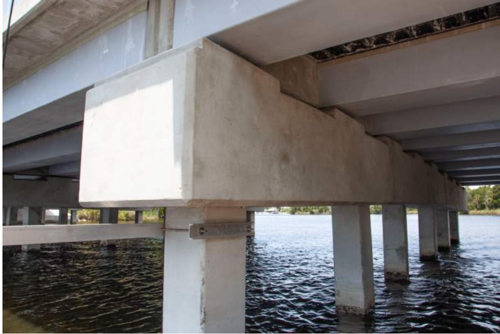
Figure 23: Span 5, looking northwest at Bent 5, view from south side
