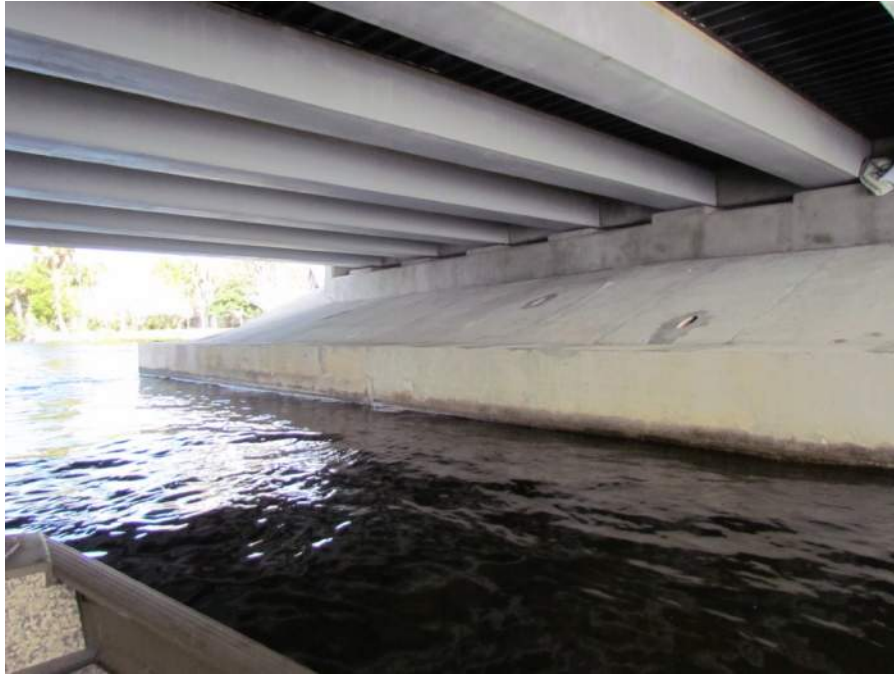
Figure 38: End Bent 6 at 3 months, looking northeast
