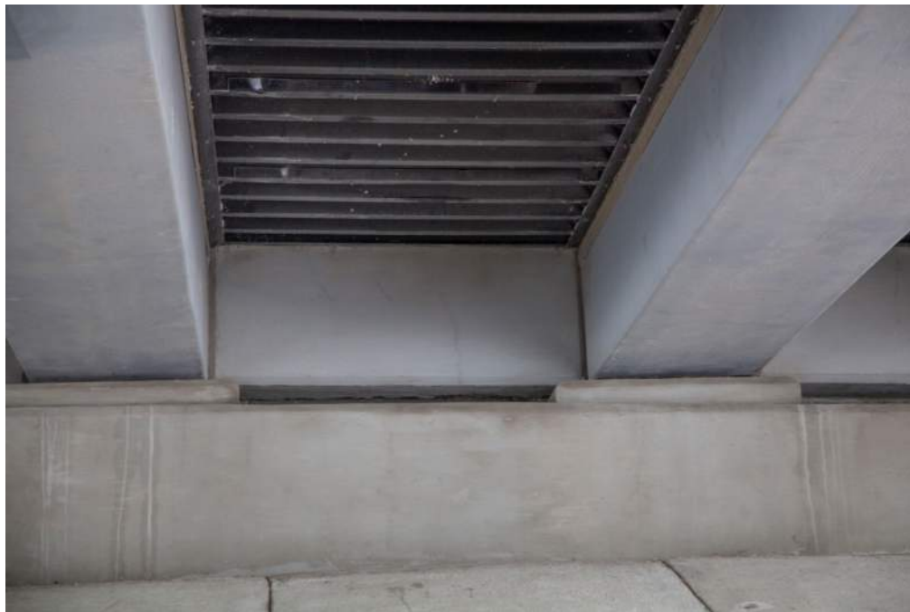
Figure 33: Diaphragm in End Bent 1 at 6 months, looking west
