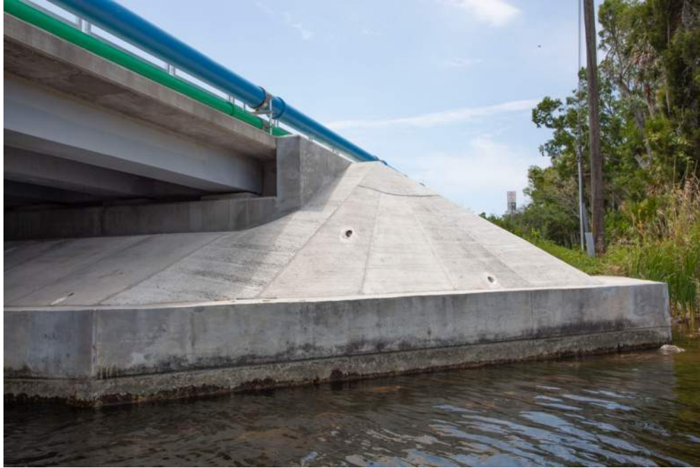
Figure 11: End Bent 1, looking west, view from north side
