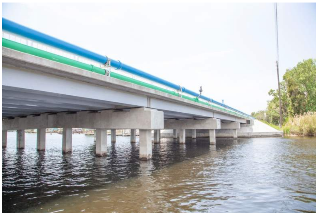
Figure 10: Spans 1-4, looking southwest, view from north side
