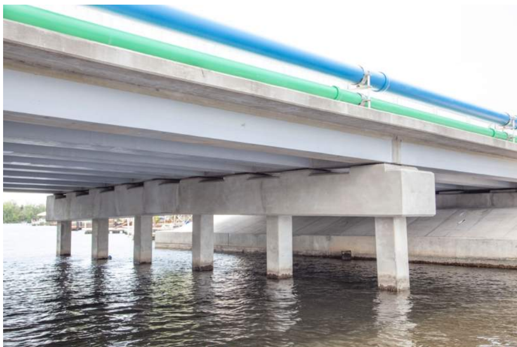
Figure 19: Span 2, looking southwest at Bent 2, view from north side
