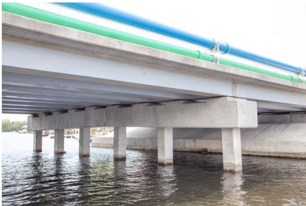
Figure 35: Bent 2 at 6 months, view from north side, looking southwest
