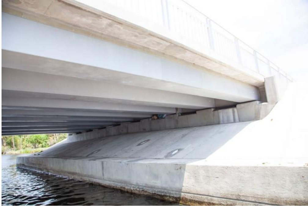
Figure 15: End Bent 6 and Span 5, looking northeast, view from south side
