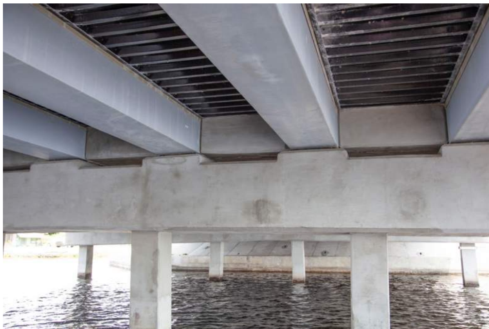
Figure 25: Span 3 underside, looking east at Bent 4
