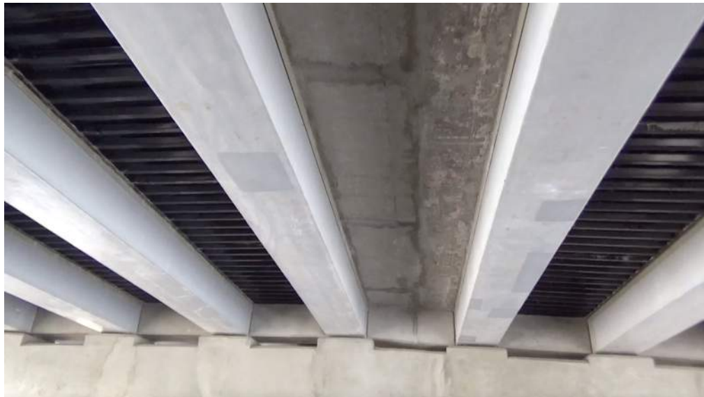
Figure 24: Span 2 underside, looking west
