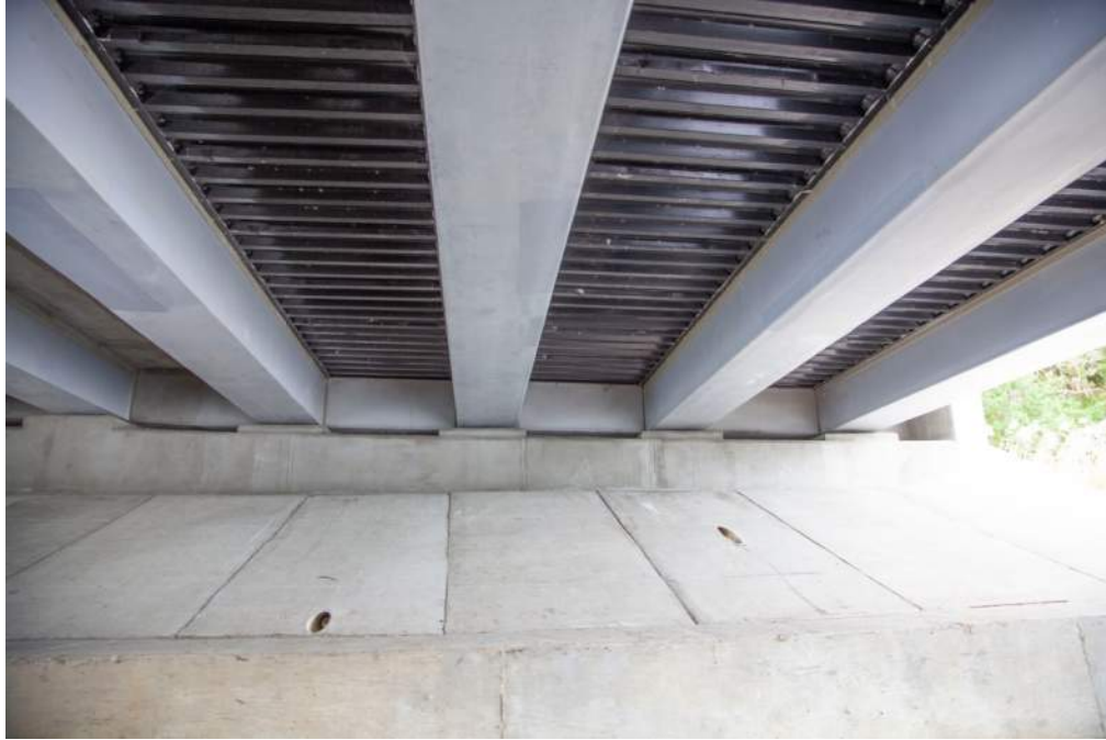
Figure 13: End Bent 1, looking west
