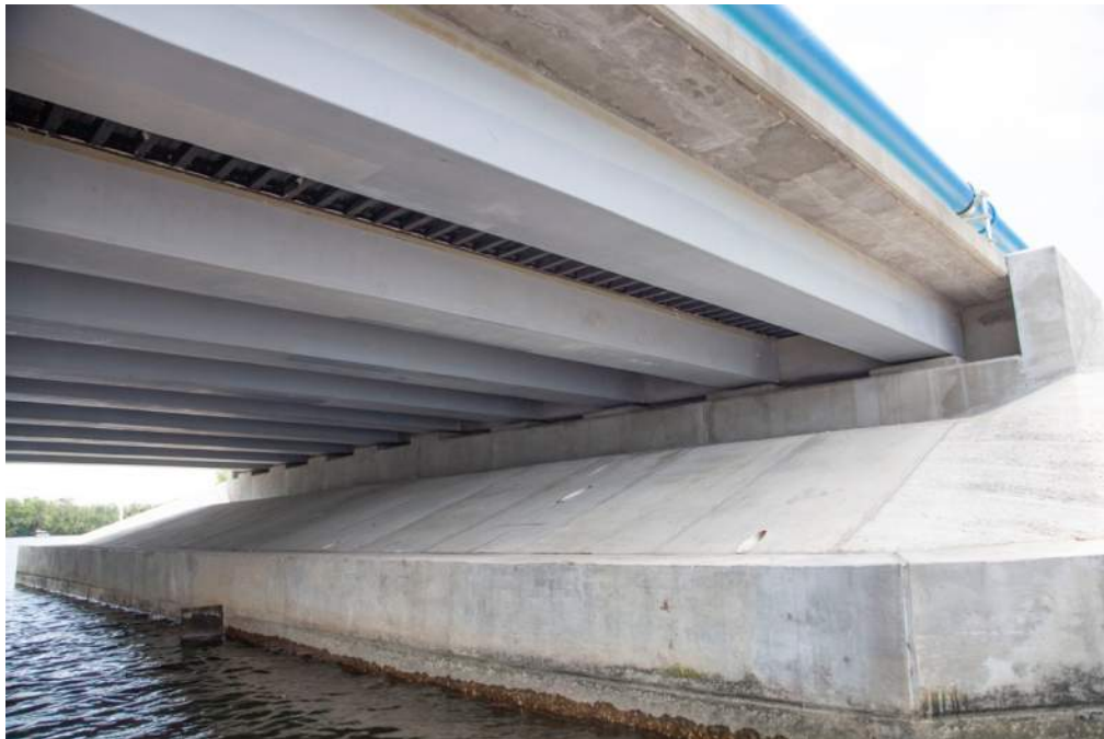
Figure 12: End Bent 1, looking southwest, view from north side
