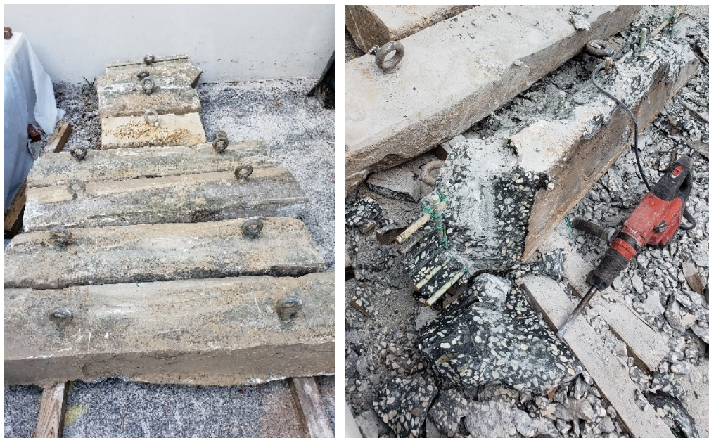
Figure 8 – (b) coring activities on test blocks, and (c) cores extracted
