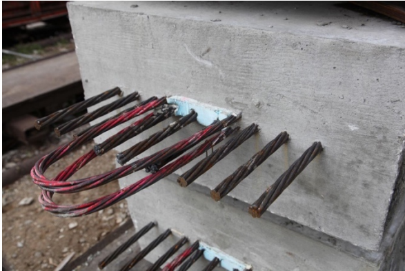
Figure 72: Steel-stranded sheet pile
