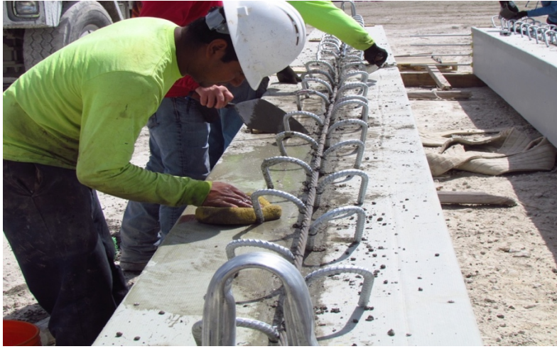
Figure 134: Finishing work on HCB
