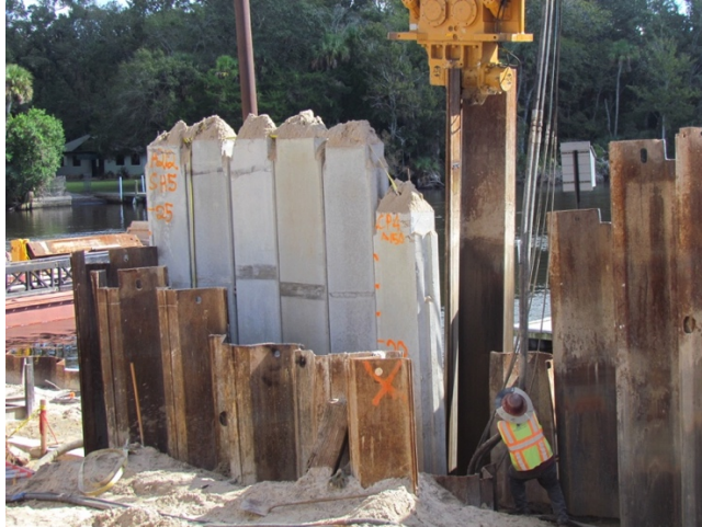
Figure 90: West side seawall (wall 6A)
