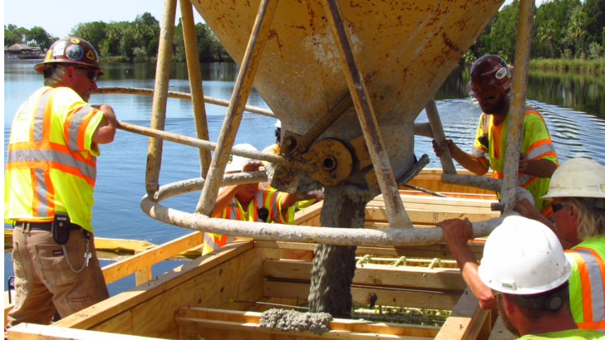
Figure 98: Casting of Bent 4 pier cap
