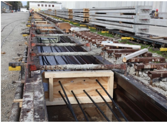
Figure 62: CFCC strands through plywood header
