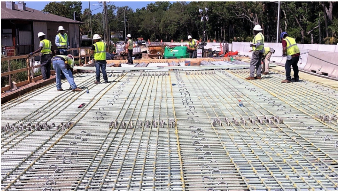
Figure 204: GFRP deck reinforcement for Phase III (Figure provided by FDOT)
