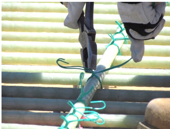
Figure 180: Tying GFRP deck reinforcement
