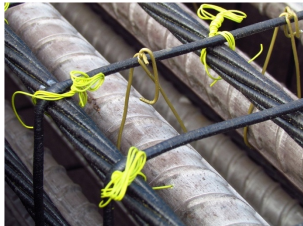
Figure 37: Wires to secure stainless steel bars
