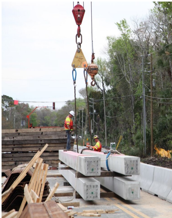
Figure 4: Cables attached to CFCC piles
