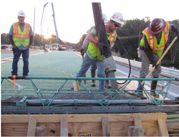
Figure 189: Pouring deck
