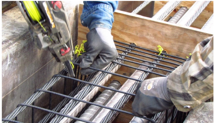
Figure 35: Tying CFCC spirals
