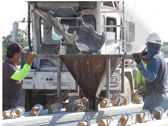
Figure 166: Hopper used to fill HCBs
