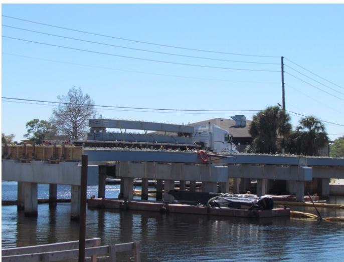
Figure 149: Beams arriving at Halls River Bridge
