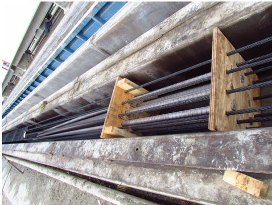
Figure 34: Stainless steel bar installation
