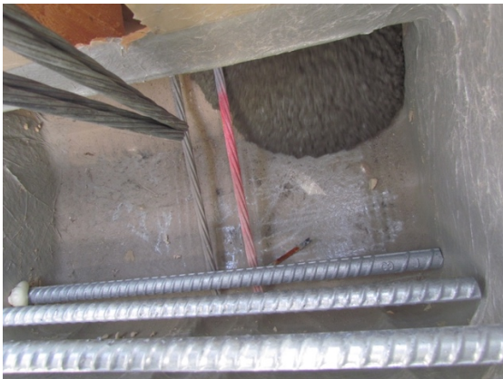
Figure 167: Filling of HCB chimney with SCC Figure 168: Filling of HCB chimney with SCC
