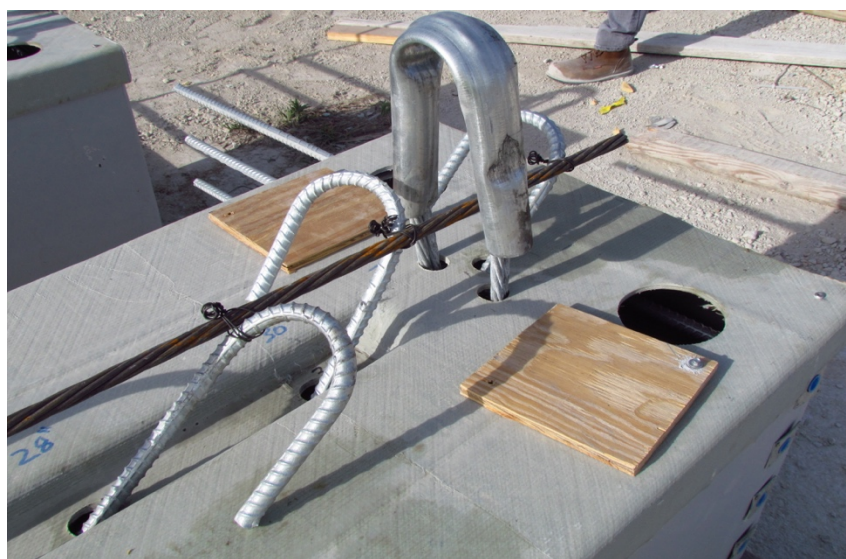
Figure 130: Plywood squares to cover SCC fill holes
