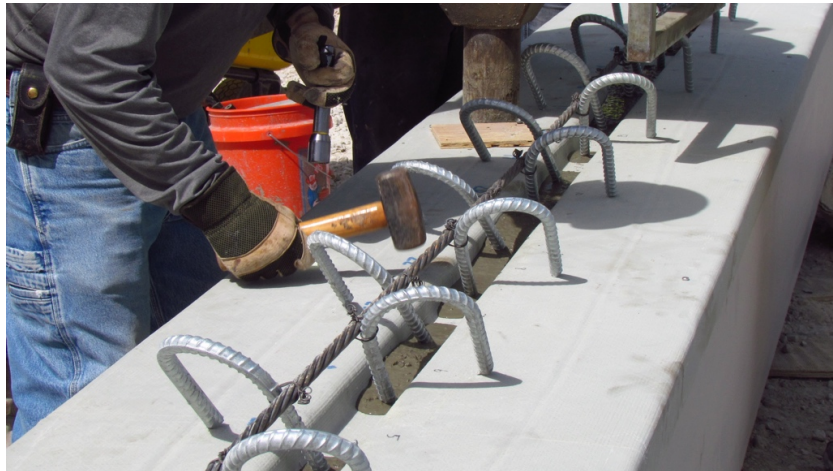
Figure 132: Mallet used to strike FRP lid
