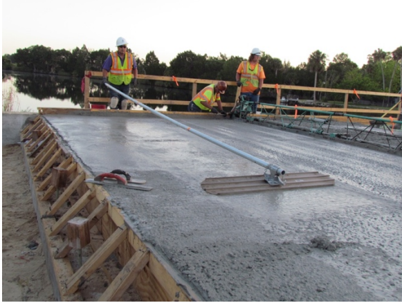
Figure 192: Bull float poured concrete
