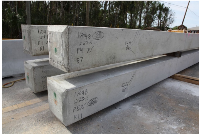
Figure 2: CFCC piles stored at Halls River Bridge
