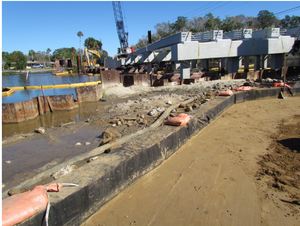
Figure 81: West side sheet pile walls (1A, 2A, and 3A)
