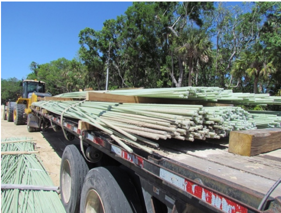
Figure 178: GFRP bars stored on trailer
