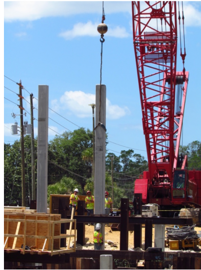
Figure 15: Cutting Bent 1 Pile 2
