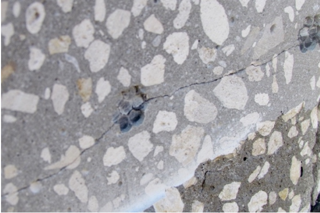
Figure 8: Pile R13 cutoff recessing of strands
