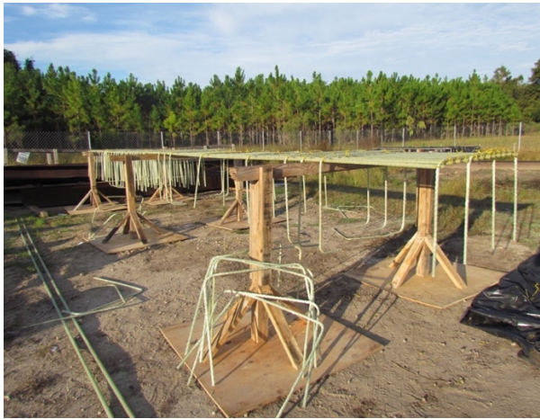
Figure 104: Wood stands for GFRP
