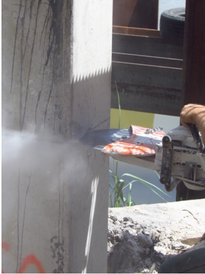
Figure 14: Cutting Bent 1 Pile 1
