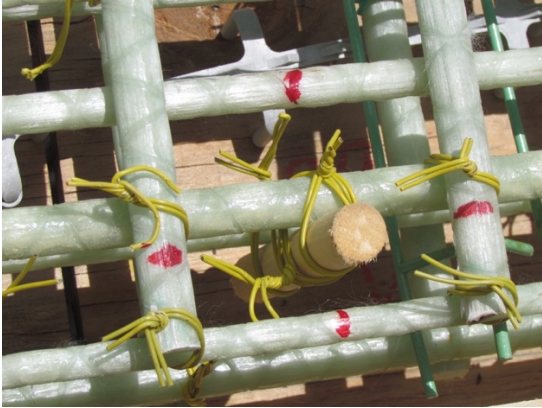
Figure 186: Wooden dowel installation
