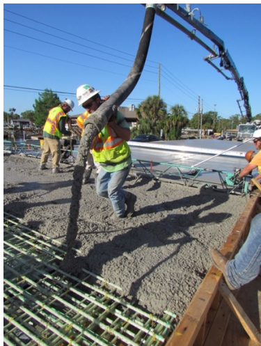
Figure 196: Pumping of deck concrete
