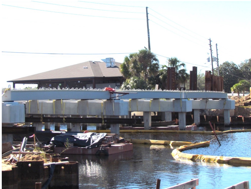
Figure 147: HCBs installed
