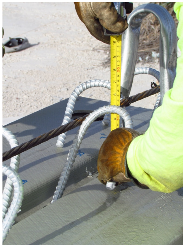
Figure 128: Placement of shear connectors
