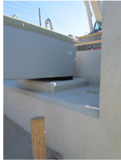
Figure 157: Installed beam on bearing pad
