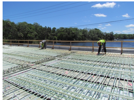
Figure 181: Tying GFRP deck reinforcement
