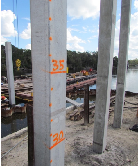
Figure 53: CFCC piles at Bent 1
