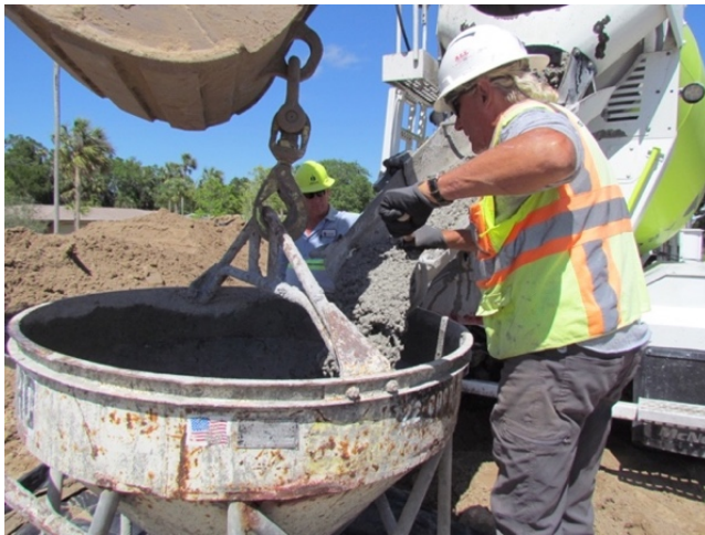
Figure 175: Bucket filling with RCA concrete
