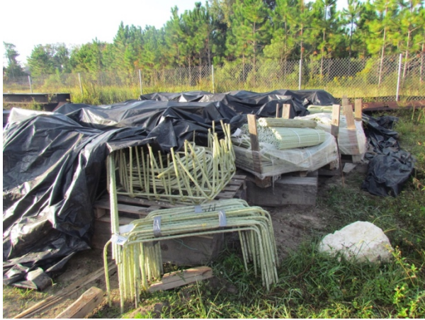
Figure 102: GFRP at storage yard
