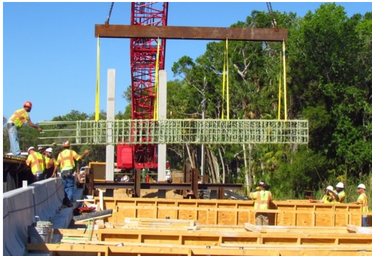
Figure 95: Installation of GFRP pier cap cage
