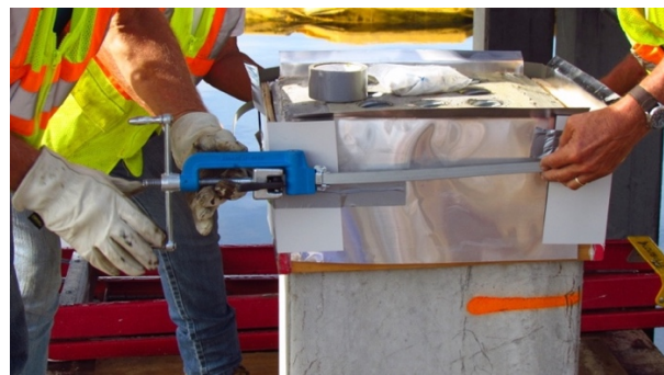
Figure 47: Securing of metal flashing
