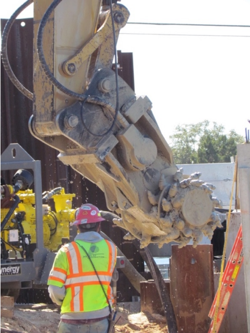
Figure 79: Trencher for CAT336E
