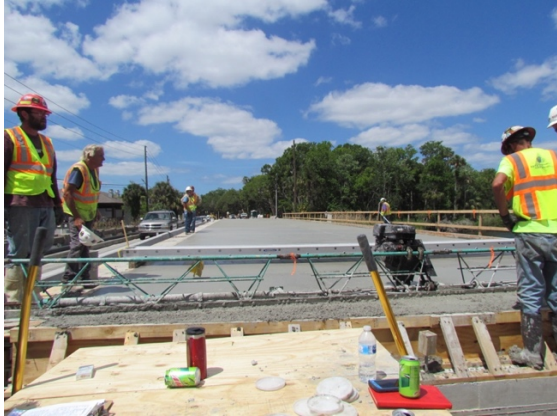
Figure 198: Finish screeding deck
