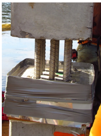
Figure 48: Dry-fit of splice pile
