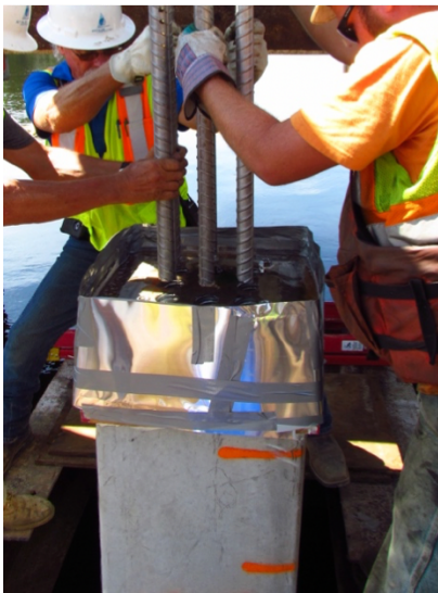
Figure 49: Placement of splice pile
