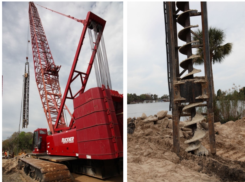
Figure 3: Crane lifting 22-inch auger; Tip of 22-inch auger
