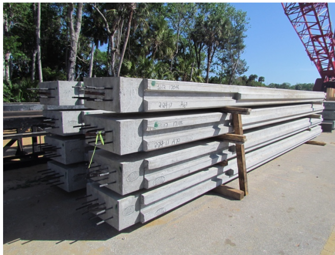
Figure 71: Storage of CFCC sheet piles at Halls River
