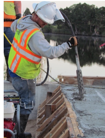
Figure 190: Vibrating concrete
