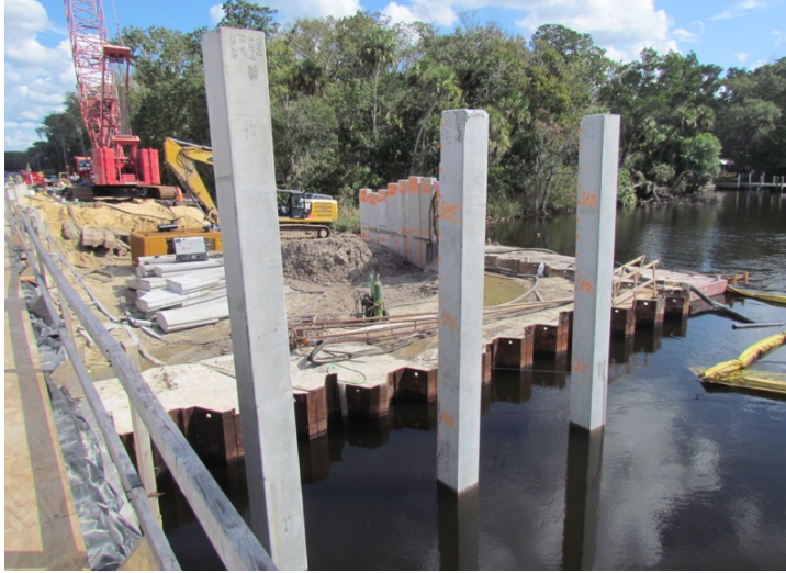
Figure 57: CFCC piles at Bent 5
