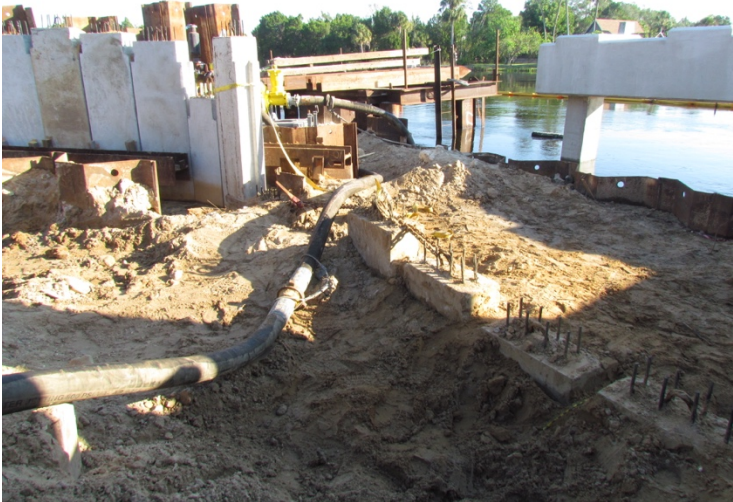
Figures 78: Sheet piles (West HRB)
