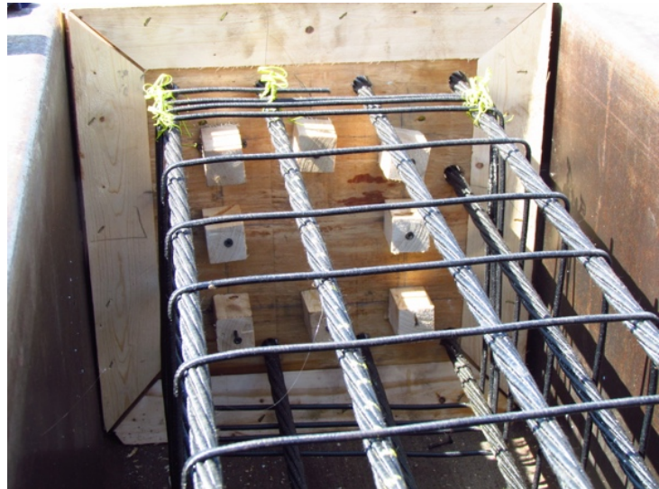
Figure 39: Blocks to secure metal tubes and bars
