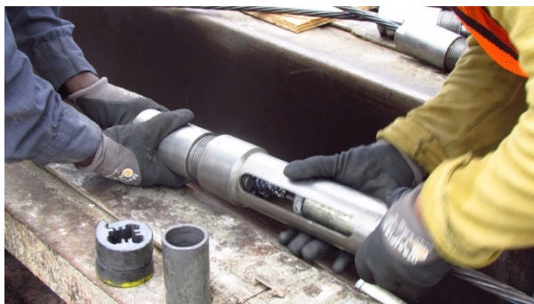
Figure 26: CFCC-steel coupler installation
