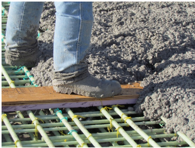
Figure 194: Block-out during pour
