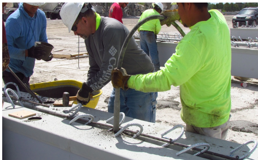
Figure 133: Vibrator used to aid in concrete flow
