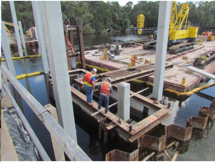
Figure 54: CFCC piles at Bent 2
