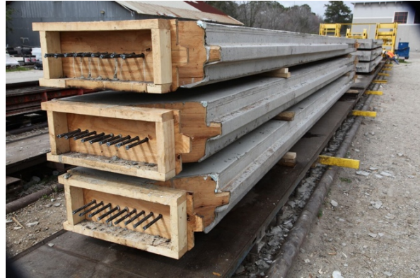
Figure 73: Steel-stranded sheet pile in storage
