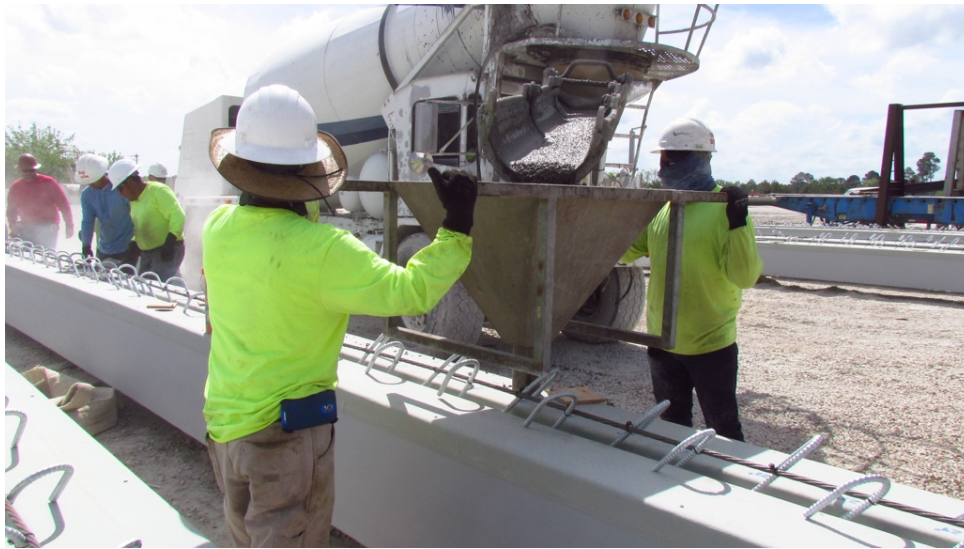
Figure 131: Hopper used to fill HCB
