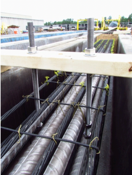
Figure 40: Lifting rod placement
