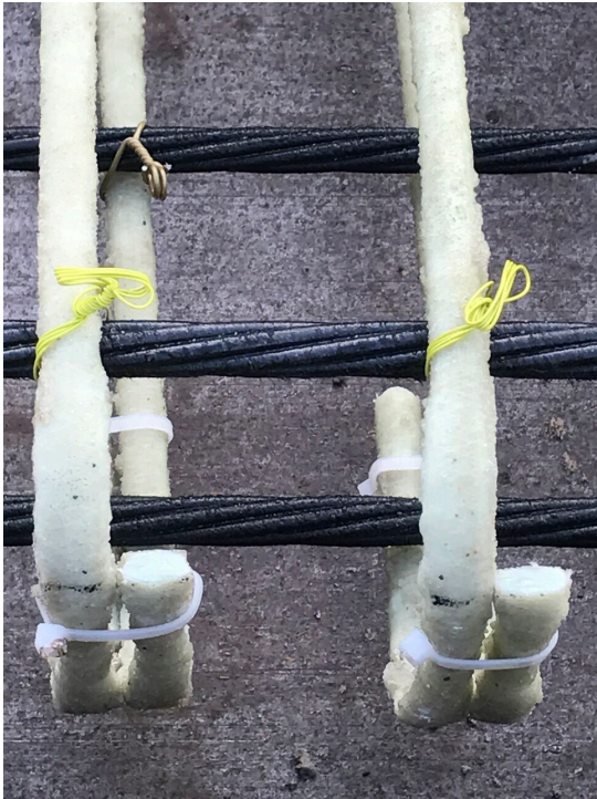
Figure 67: Ties used to secure GFRP stirrups to CFCC strands
