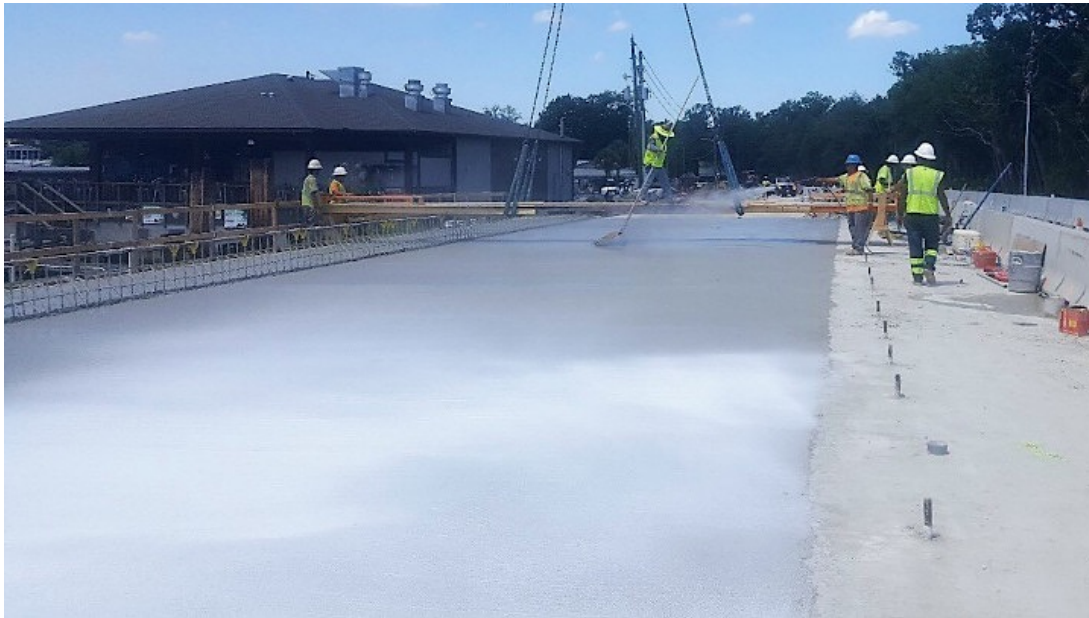
Figure 205: Complete deck for Phase III (Figure provided by FDOT)
