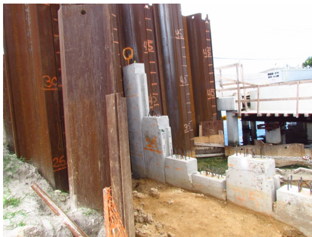
Figure 76: Installed CFCC sheet piles
