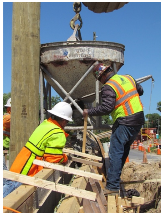
Figure 176: Pouring RCA concrete
