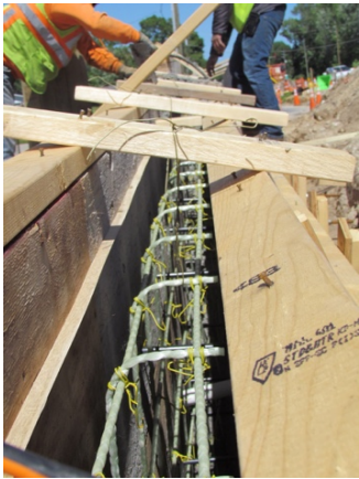
Figure 174: GFRP of RCA gravity wall
