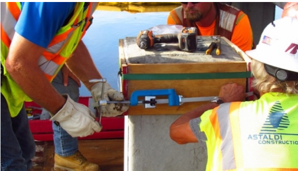
Figure 46: Tightening of plywood form
