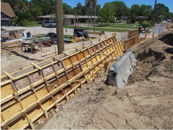
Figure 173: Formed RCA gravity wall
