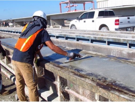
Figure 41: Pouring of SC concrete
