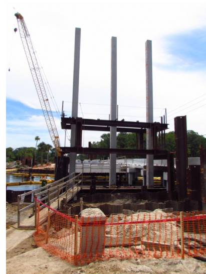
Figure 50: First splice piles at Bent 2
