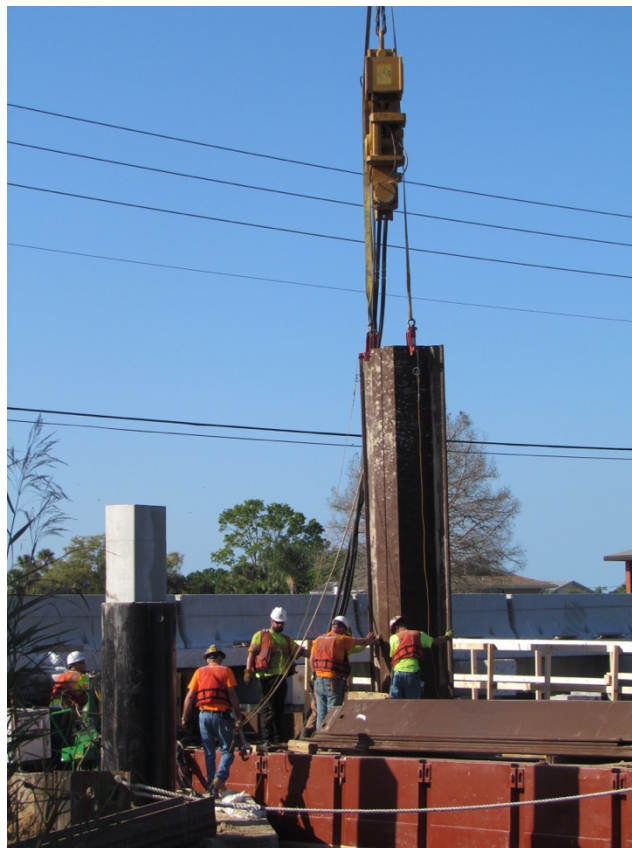
Figure 60: Temporary sheet pile installation
