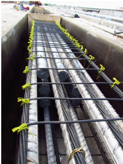
Figure 38: Installation of metal tubes
