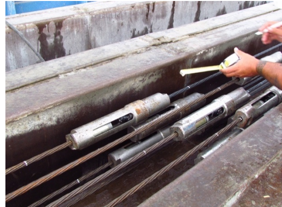
Figure 29: Coupler marked after initial stressing
