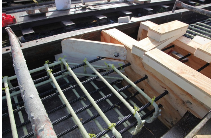
Figure 68: Tapered end of CFCC sheet pile
