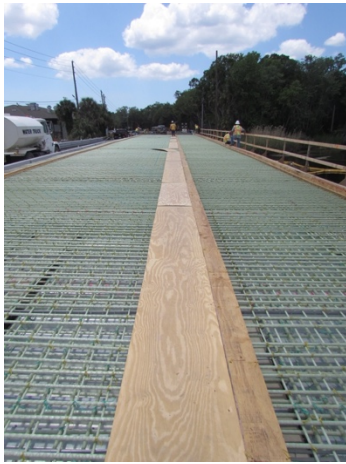
Figure 184: Plywood walkway and block-out
