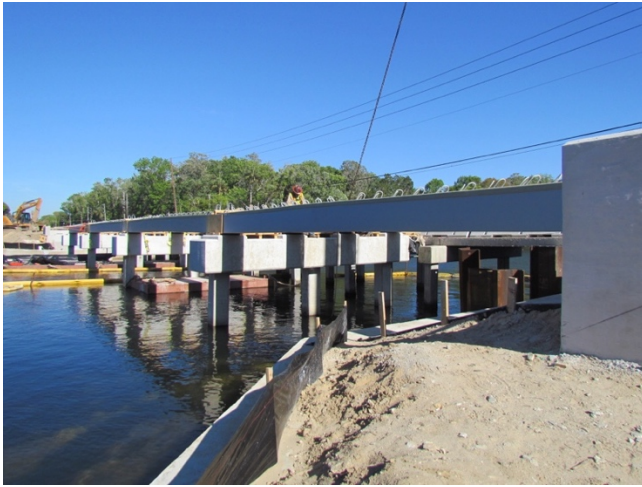
Figure 156: Installed HC Beams
