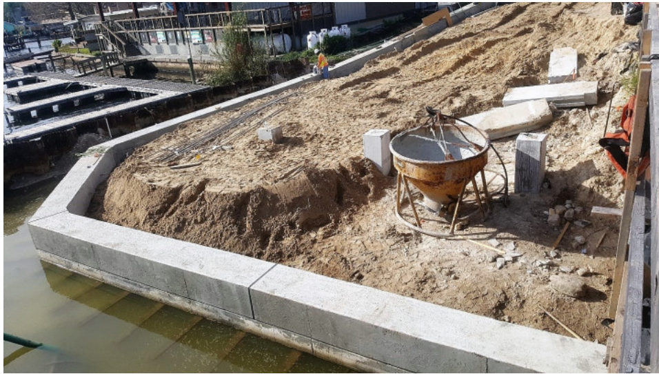
Figure 93: Sheet pile walls 4A, 5A, 6A (Figure provided by FDOT)
