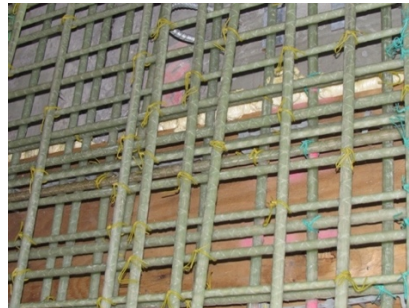
Figure 188: Spray foam in deck form
