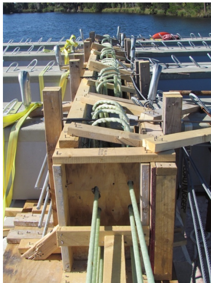
Figure 170: Reinforced and formed diaphragms
