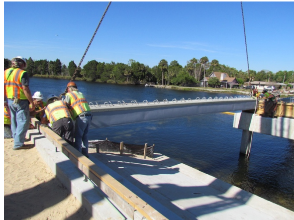
Figure 155: HC Beams being installed
