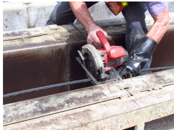
Figure 23: Cutting of CFCC strand
