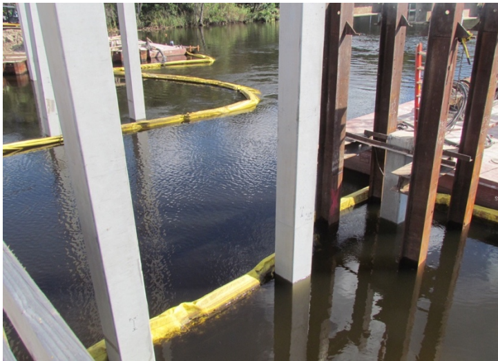
Figure 55: CFCC piles at Bent 3
