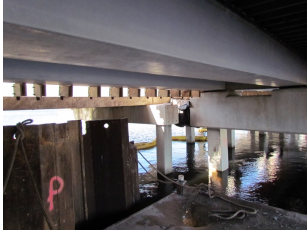
Figure 61: Demolition on existing bridge (eastbound lane)
