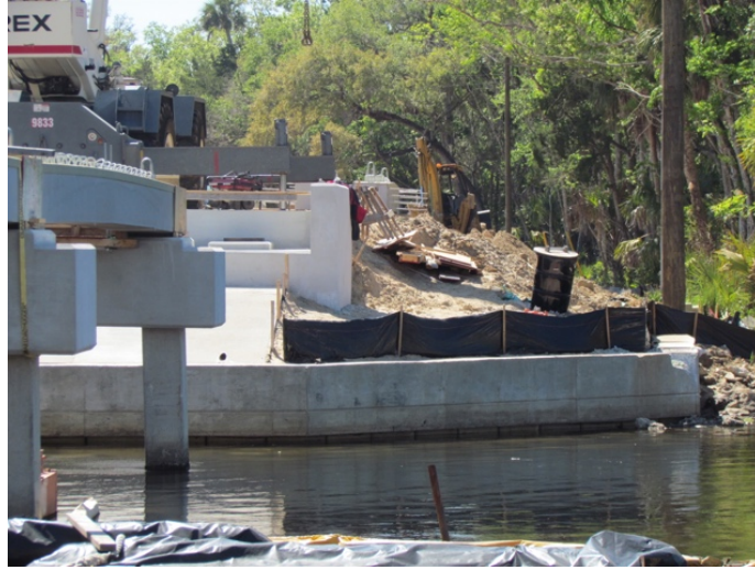
Figure 83: Sheet pile walls 1A, 2A, and 3A
