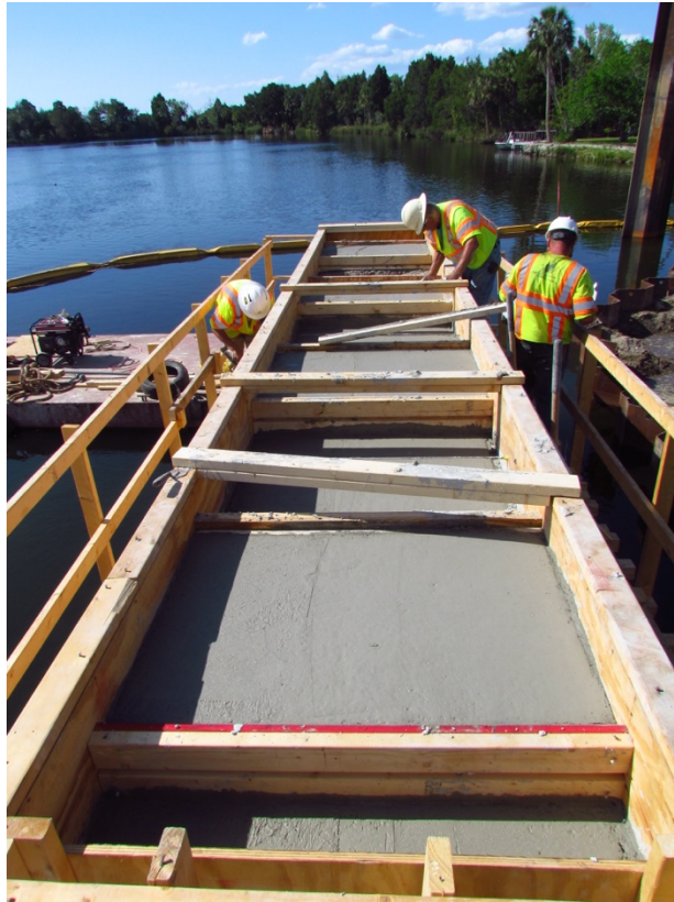
Figure 100: Completed pier cap
