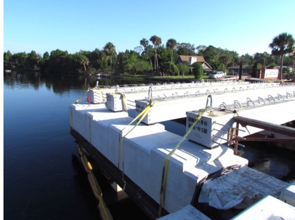
Figure 207: HCB beams strapped for Hurricane Irma
