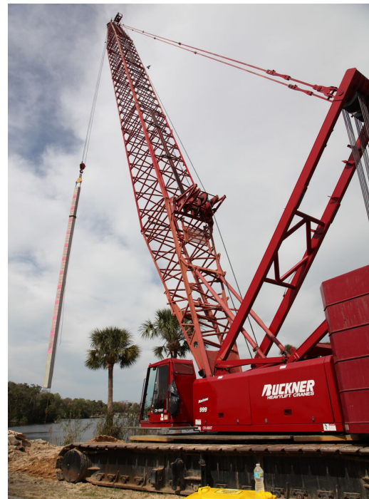
Figure 5: CFCC piles lifted by crane
