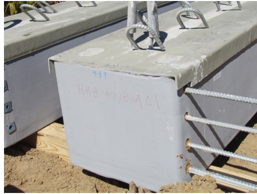
Figure 151: Unpainted beam labels on HRB-02
