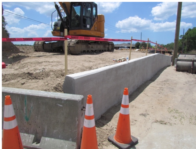
Figure 177: RCA/RAP gravity wall
