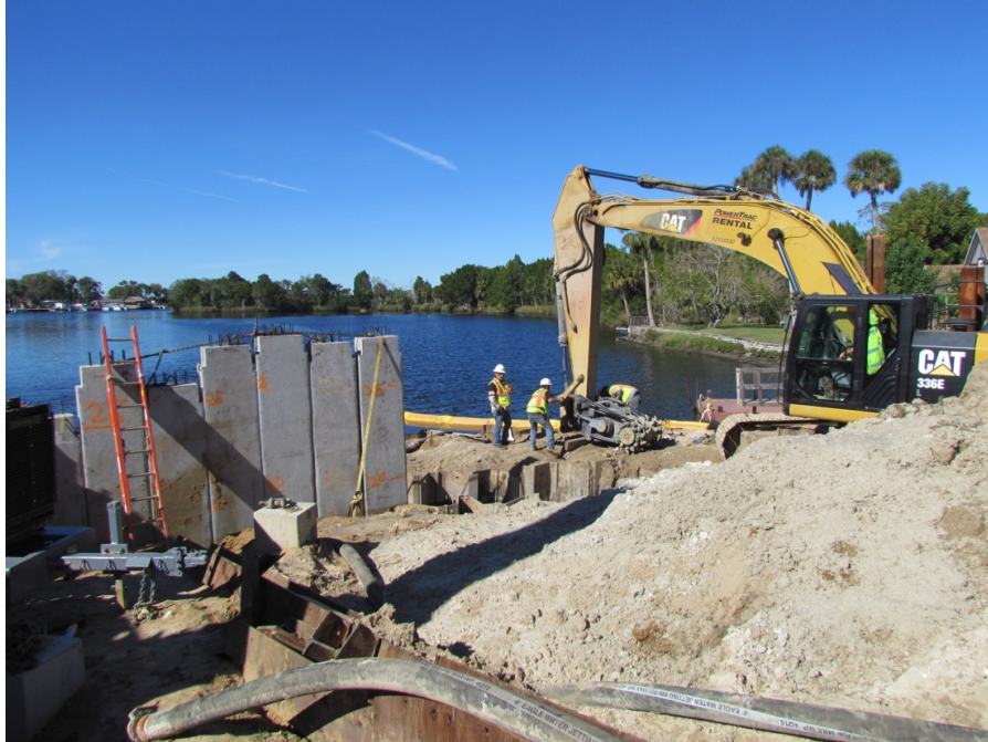
Figure 82: East side sheet pile walls
