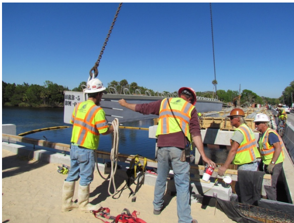
Figure 154: HC Beams being installed
