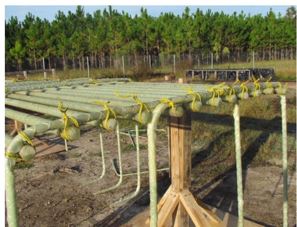
Figure 105: GFRP pier caps
