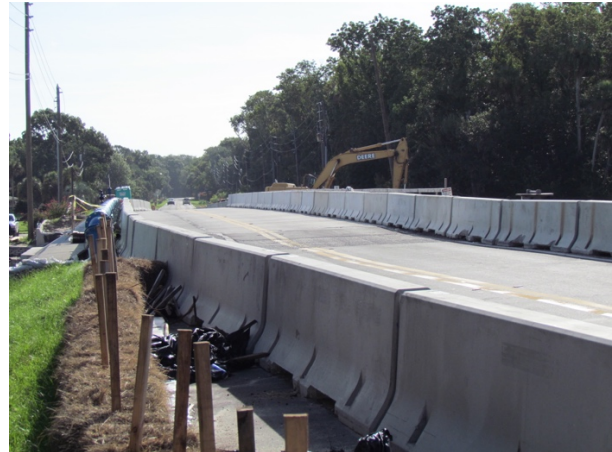
Figure 201: Completed westbound lane
