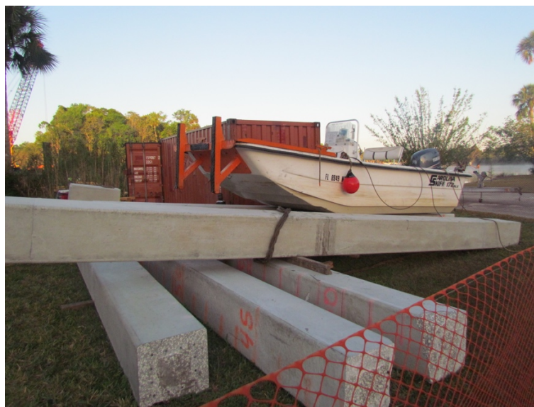
Figure 6: Stored pile cutoffs
