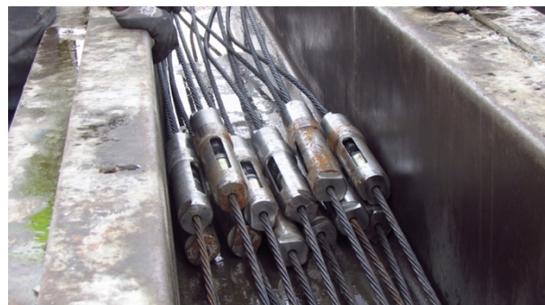
Figure 27: Aligned couplers
