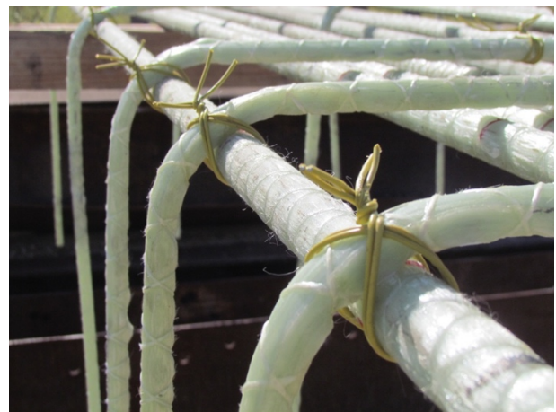
Figure 107: Plastic coated tie wires
