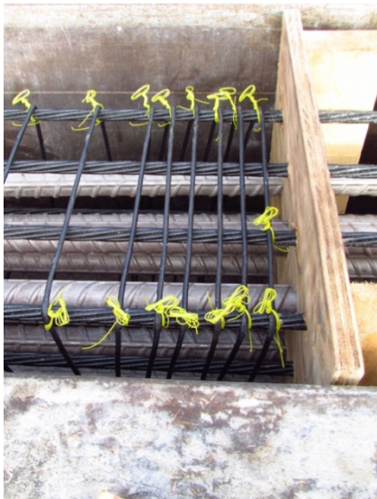
Figure 36: Tied CFCC spirals
