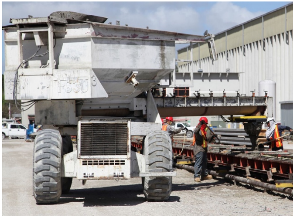
Figure 69: Placing SCC with hopper
