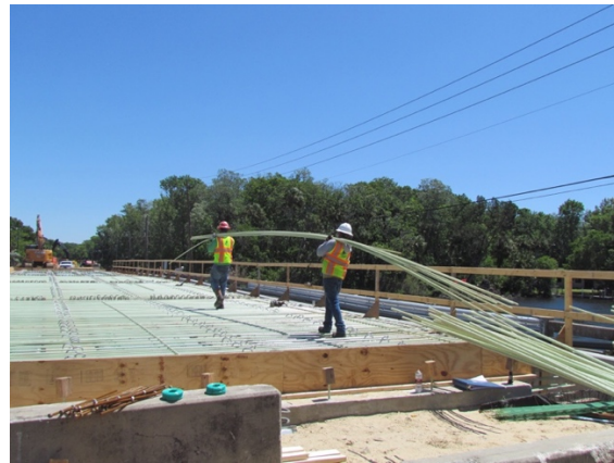
Figure 179: Workers carrying GFRP bars
