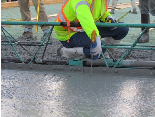
Figure 191: QC checking depth of deck
