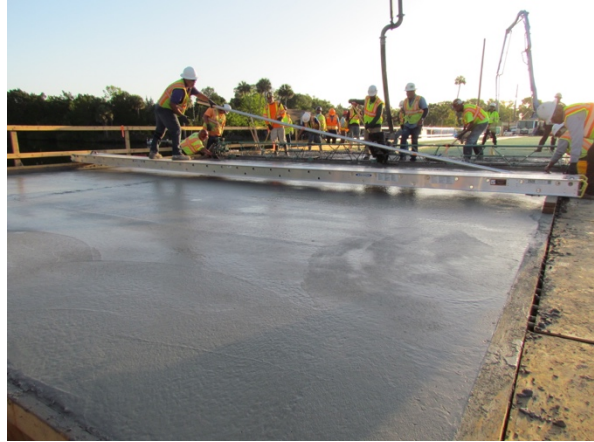
Figure 193: Concrete with smooth finish
