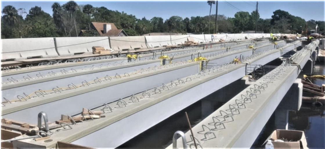
Figure 169: Phase III installed HCBs (Figure provided by FDOT)
