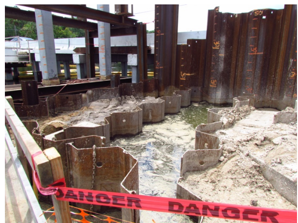
Figure 77: Double layer of metal sheet piles
