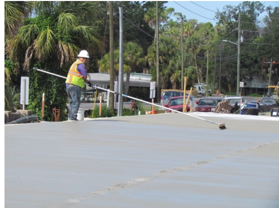
Figure 199: Broom finish to deck
