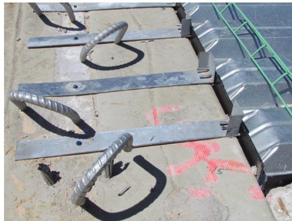
Figure 183: SIP deck form support bars
