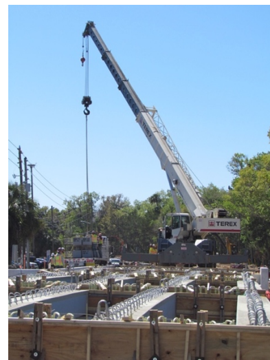
Figure 150: Beams lifted using crane
