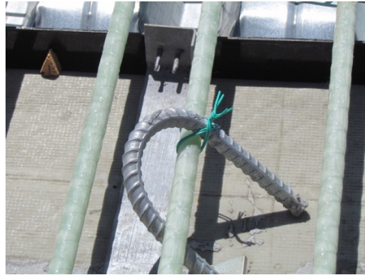
Figure 182: GFRP bars tied to shear connector
