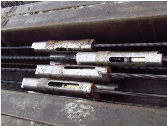
Figure 30: Coupler positions after initial stressing
