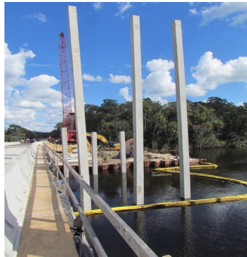
Figure 56: CFCC piles at Bent 4
