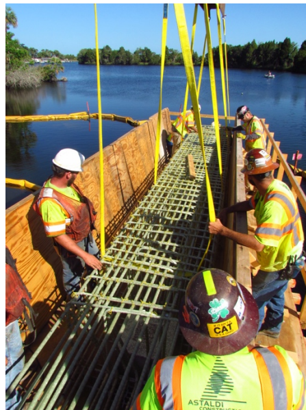
Figure 96: Crew members positioning GFRP cage
