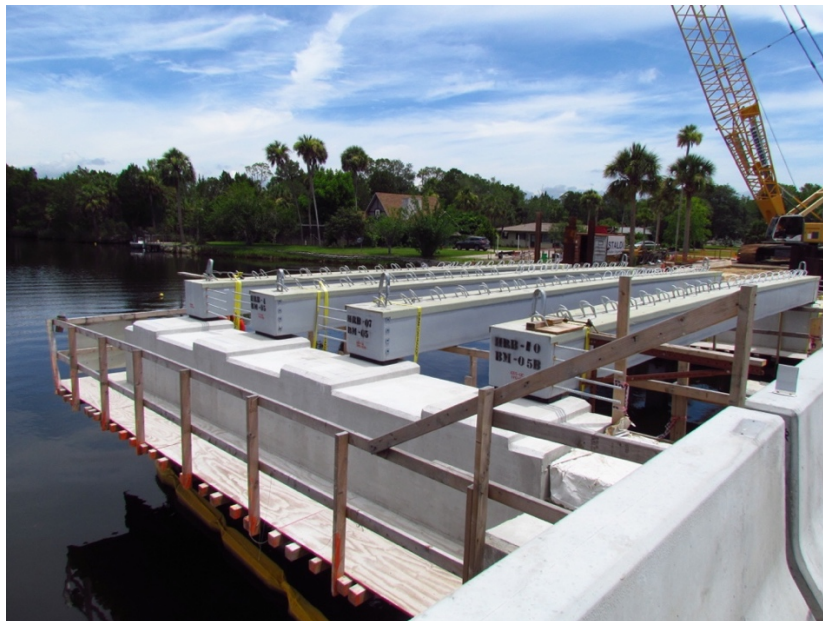
Figure 135: HCB Beams between Bents 4 and 5
