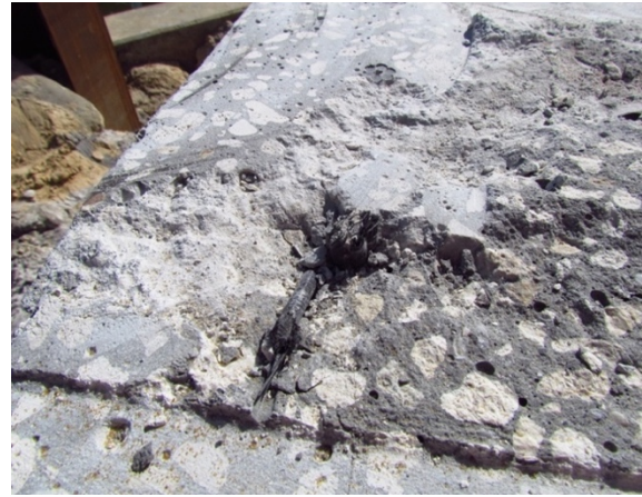
Figure 19: Recessing of CFCC (Bent 1 Pile 3)
