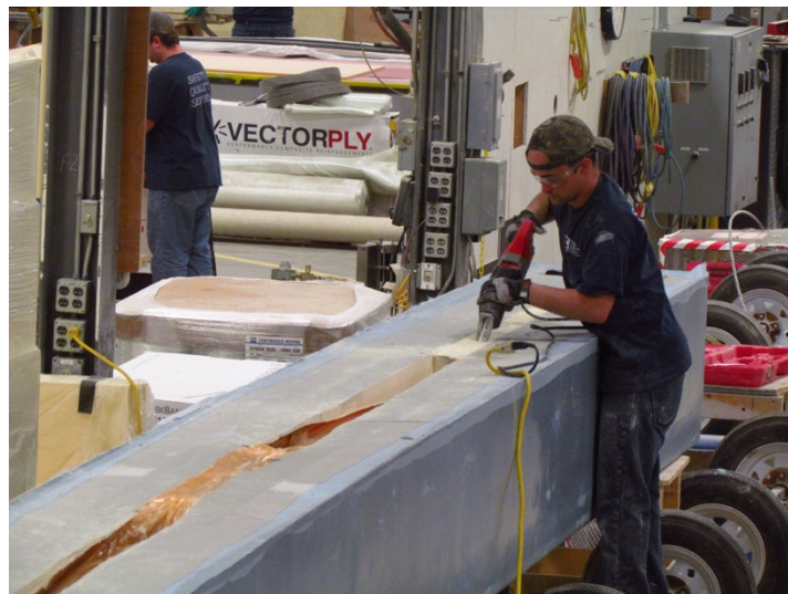
Figure 121: Cutting 4-in. channel in HCB
