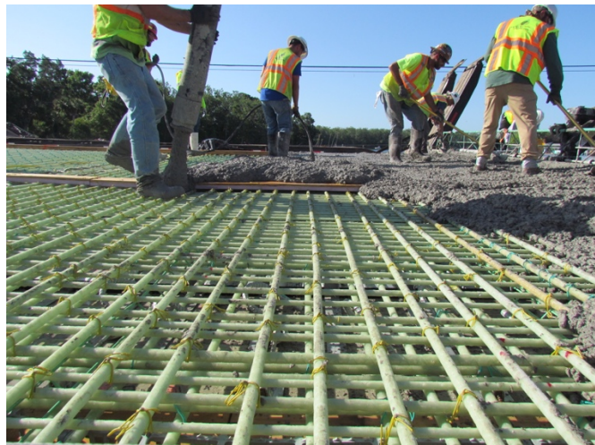
Figure 197: Tied GFRP deck reinforcement
