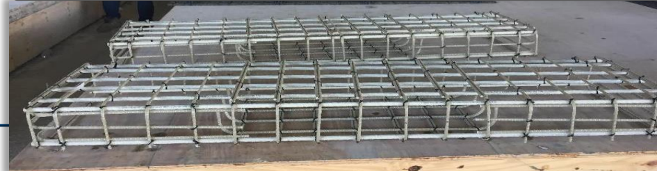
iDock pile bent caps GFRP rebar cages, Coreslab (2018)
