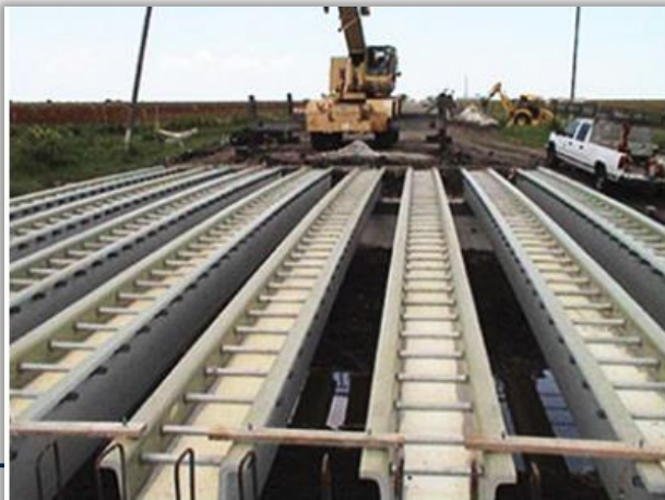
FRP girders await the next step in construction of this bridge.
