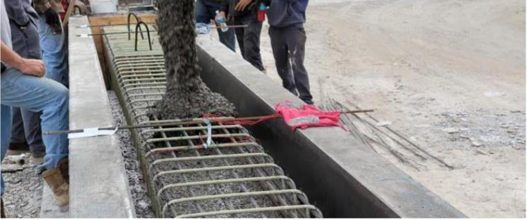
Evaluation of Glass Fiber Reinforced Polymers (GFRP) Spirals in Corrosion Resistant Concrete Piles Development of GFRP Reinforced Single Slope Bridge Rail
