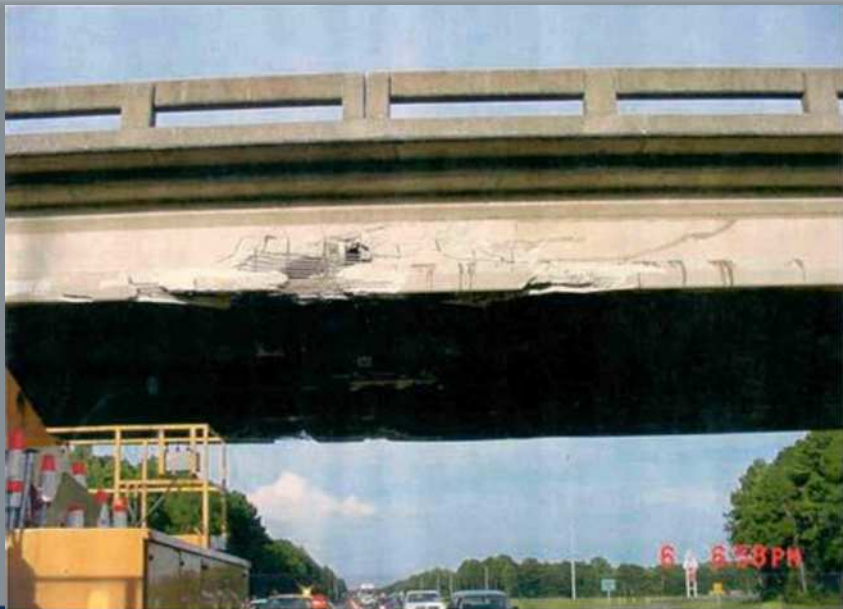
BDV31 977-01:Figure 227—Girder damage from vehicle impact in July of 2001
