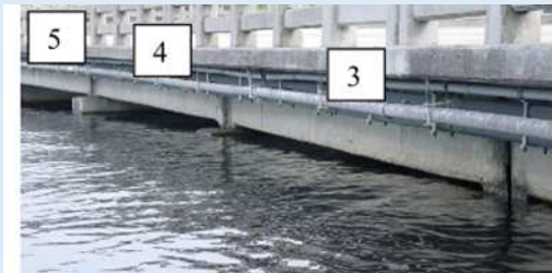
Report: BDV31 977-01 (University Blvd Bridge, 2011)
