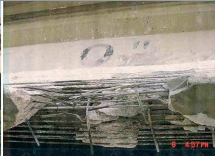
BDV31 977-01:Figure 227—Girder damage from vehicle impact in July of 2001
