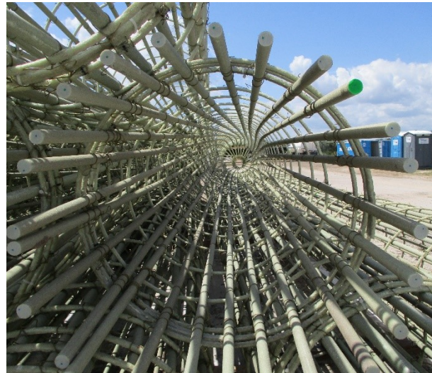
GFRP Secant-Pile Shaft cages for A1A-Flagler Beach seawall (2019)
