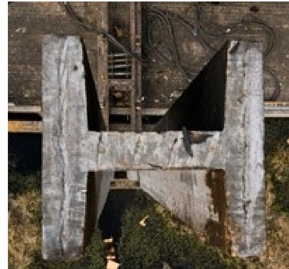
UHPC-PC H-Pile for CR-339 demonstration (2020)
