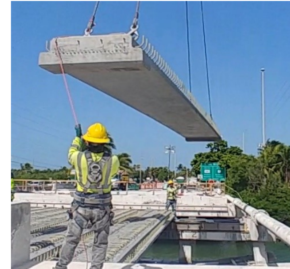
CFRP-PC FSB's US-1/Cow Key span replacements (2020)
