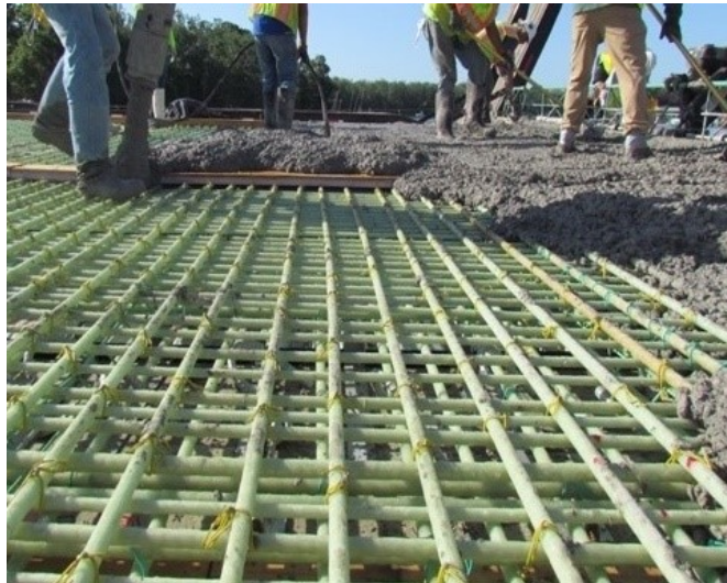
GFRP rebar for deck & substructure of Halls River Bridge (2017-18)
