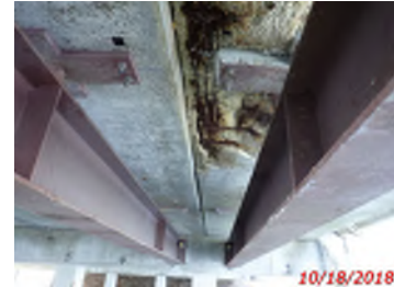
Underpinning at midspan
