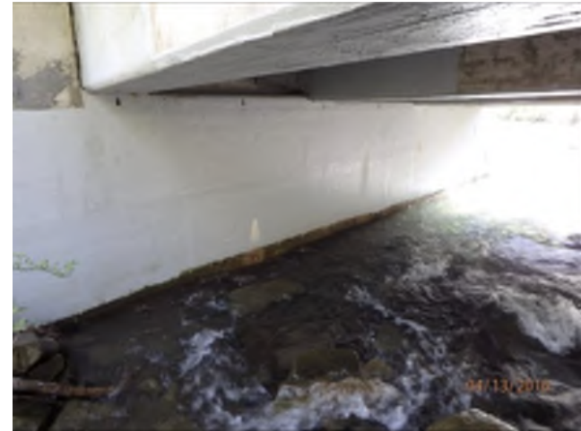
CFRP wraps in abutments and underside of a T-beam
