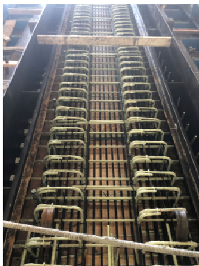
CFRP prestressing & GFRP rebar inside form
