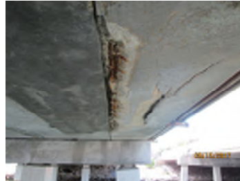
Exposed reinforcing, spalling, cracking & delamination
