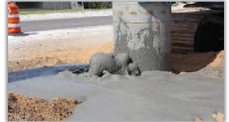
Secant-Pile alignment and auger drilled soil removal, prior to concrete grouting
