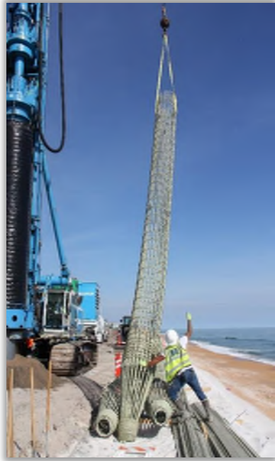
1847 Secant-Piles were installed in only 4-1/2 Months for SR-A1A
