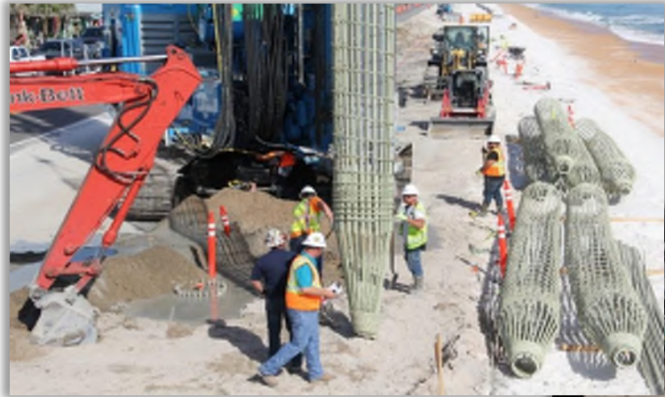
Site assembled GFRP Cage-installations, at Flagler Beach, Florida
