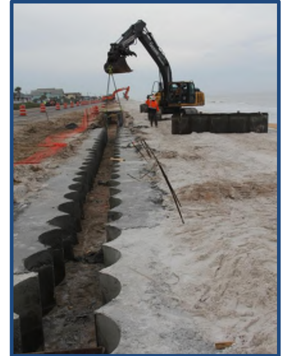
Removal of steel formwork, prior to drilling Secant-Piles
