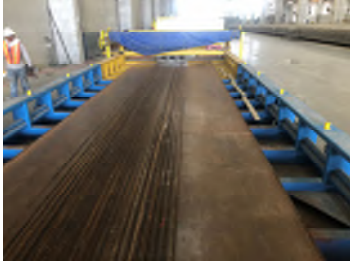
CFRP prestress in casting bed
