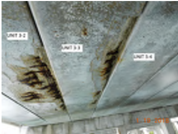
Exposed reinforcing, spalling, cracking & delamination
