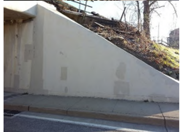
GFRP Wrapping on a headwall and a wing wall
