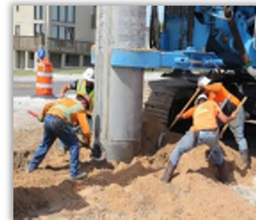
Secant-Pile alignment and auger drilled soil removal, prior to concrete grouting
