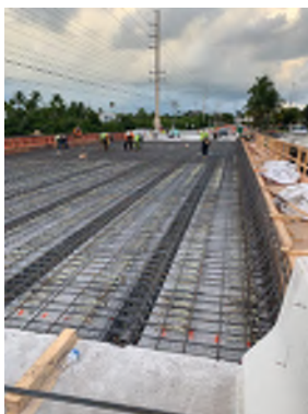
Deck Reinforcing Installation
