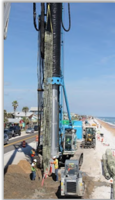
1847 Secant-Piles were lifted, aligned, centered, and lowered into position
