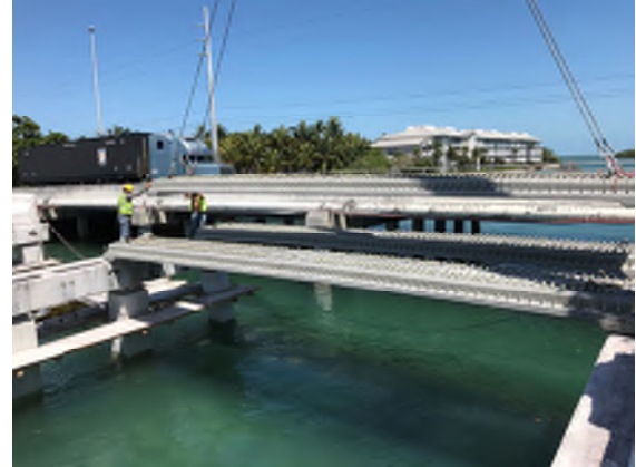
Erection of 3 rd FSB
