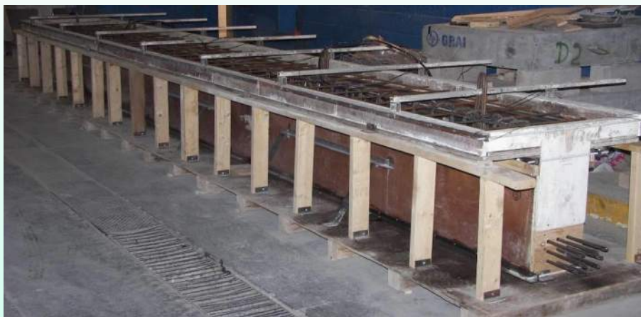
Reinforcing Cage and Concrete Casting
