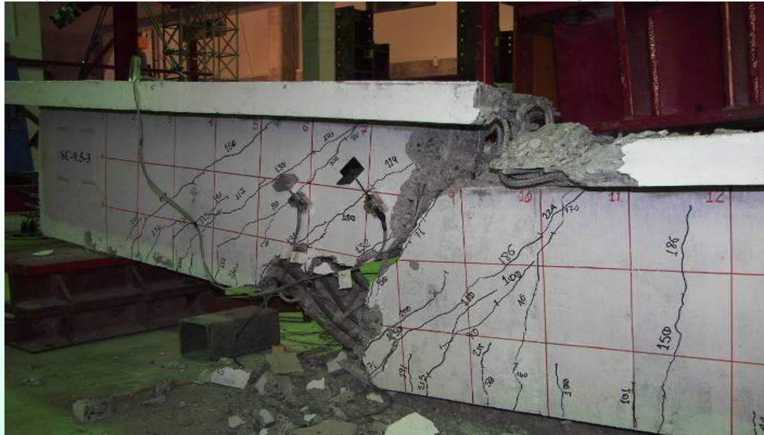
Shear Failure of SC-9.5-3 (CFRP @ d/3 )
