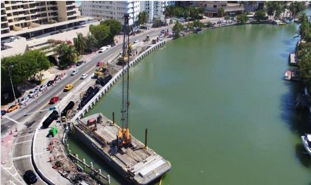
Miami Beach seawall-bulkhead and road raising project. (Photo / Bruce Mowry, city engineer / courtesy http://gatehouseprojects.com/risingseas/home/site/news-jrnl.com )
