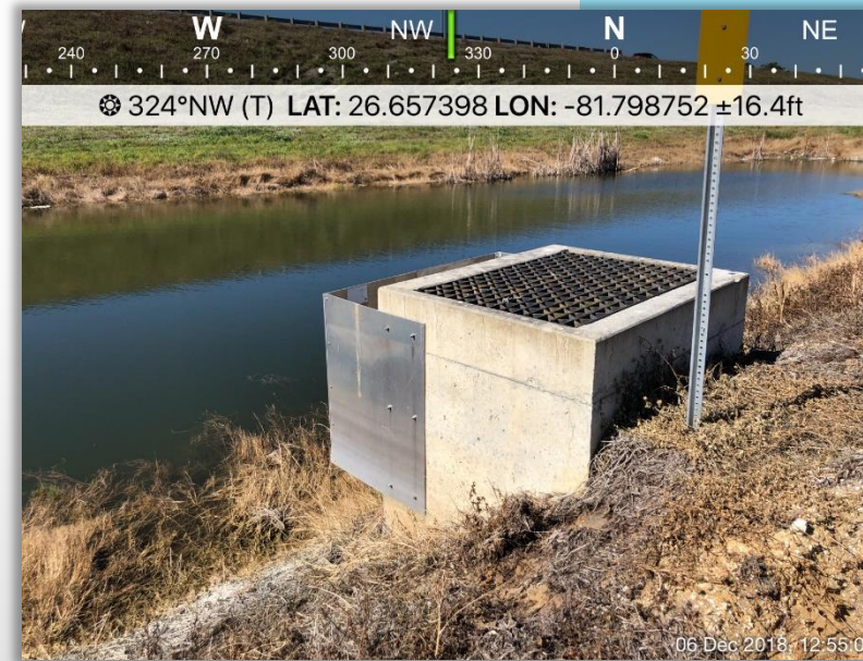
(a) Plan view locations of 3 retention pond overflow structures; (b) Photograph of structure CS-2.
