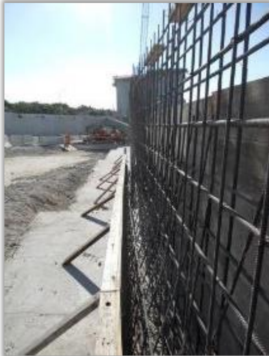
Wall 6 under construction & Typical Cross-section of Retaining Walls 5 and 6
