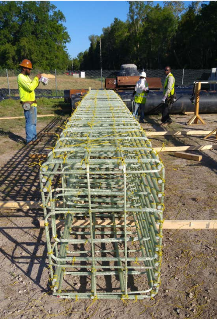
PHOTO: GFRP cage assembly for the Halls River Bridge Project, April 2017.
