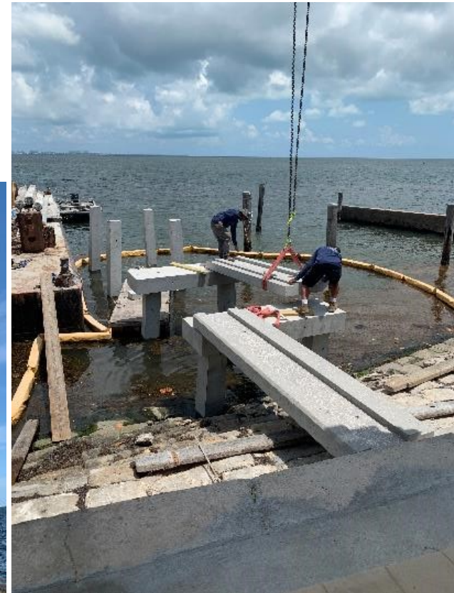
Precast Slab-Beam installed in sections after cap placement
