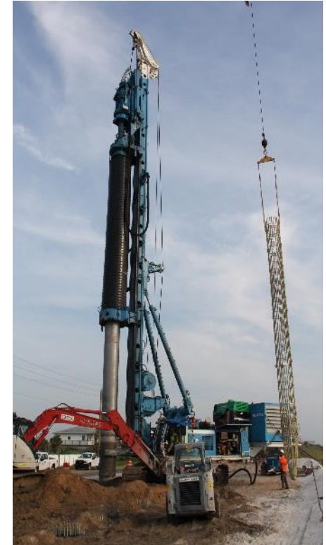
1,847 Secant-piles installed. 5,000 linear feet of pile-cap
