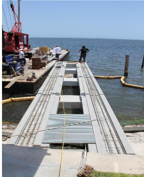
Slab-Beam with Grating
