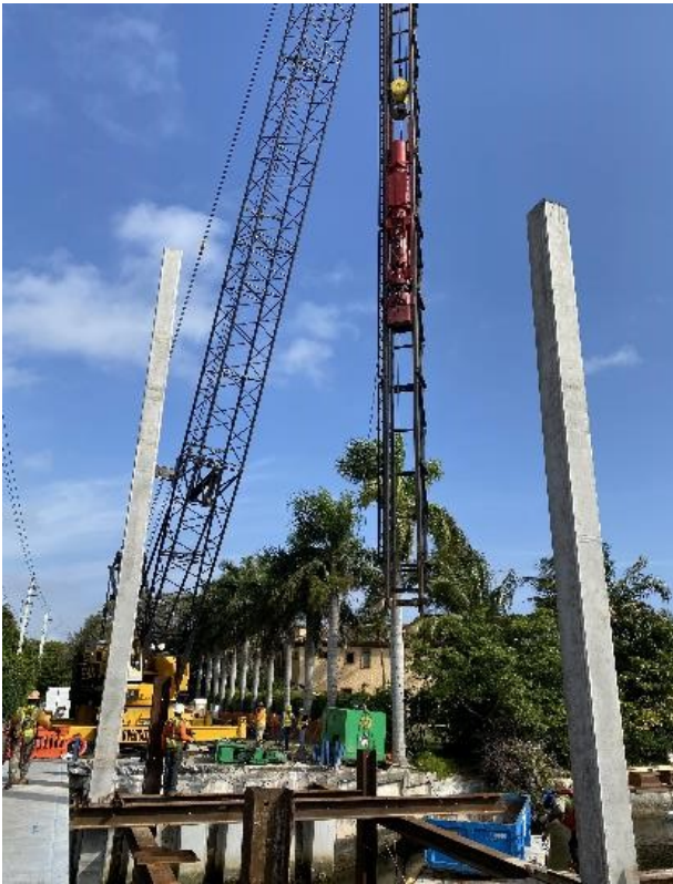
Pile alignment via template construction to allow for FDOT specified tolerances
