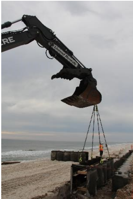
Guide wall trench boxes installed to assure pile alignment
