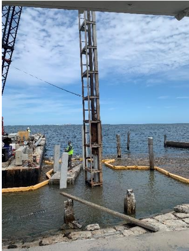
Pile-Driving at iDock
