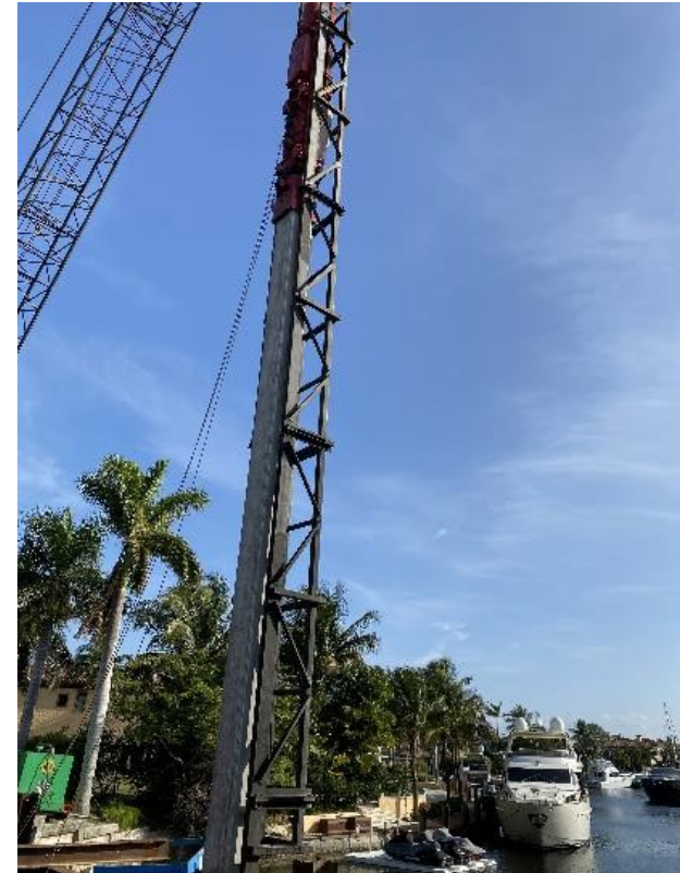
Pile installation challenging due to power lines and tight site conditions
