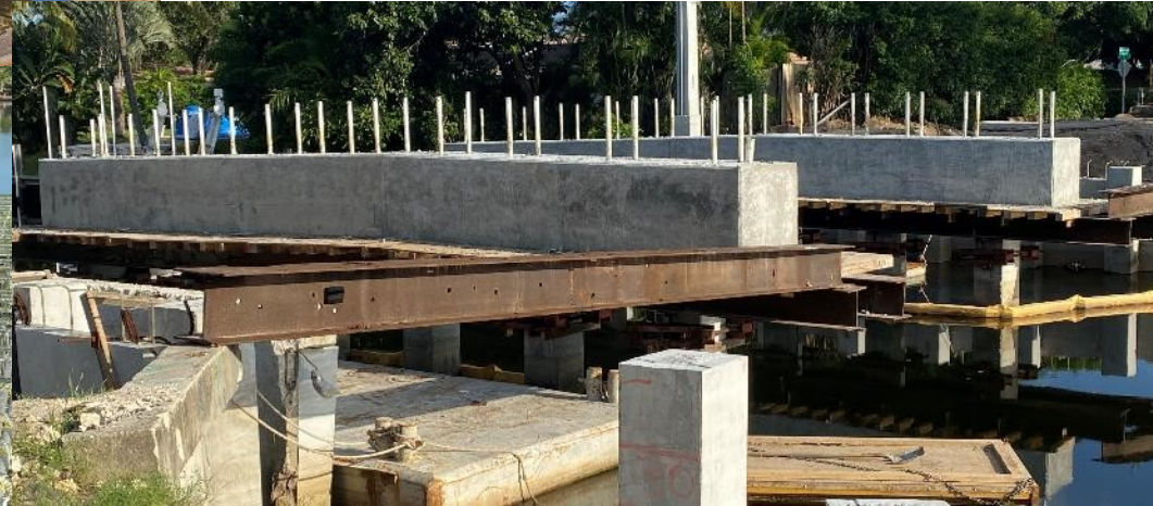
Casting completed and forms stripped
