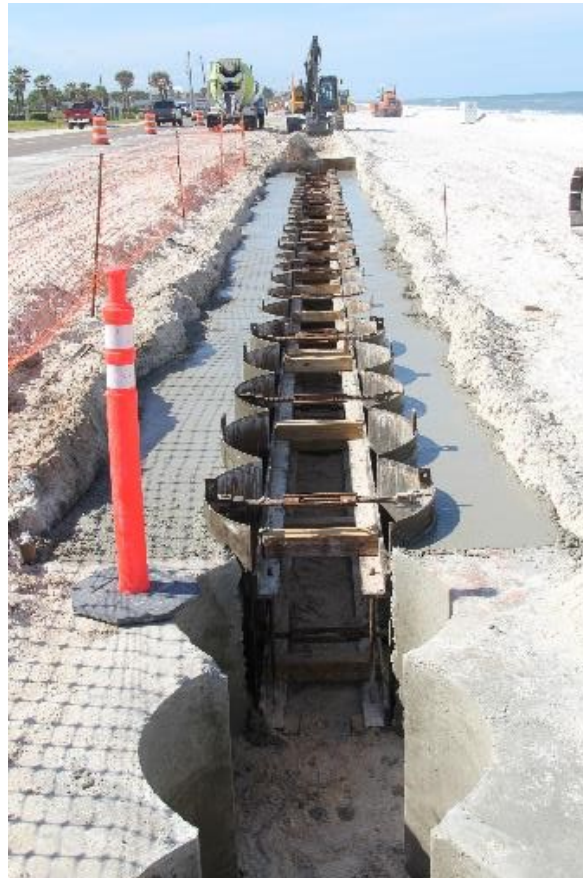
Secant-piles installed via guide wall form
