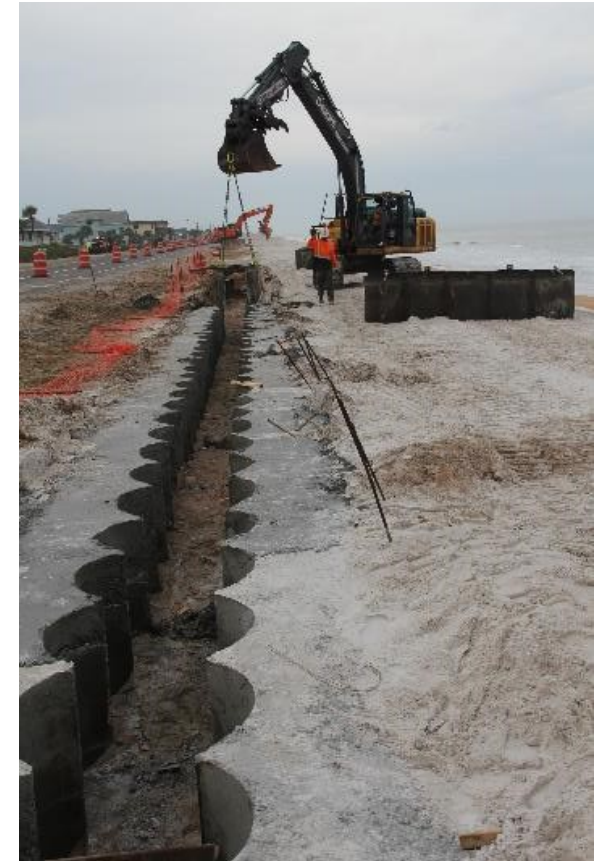
Removal of steel formwork prior to drilling secant-piles
