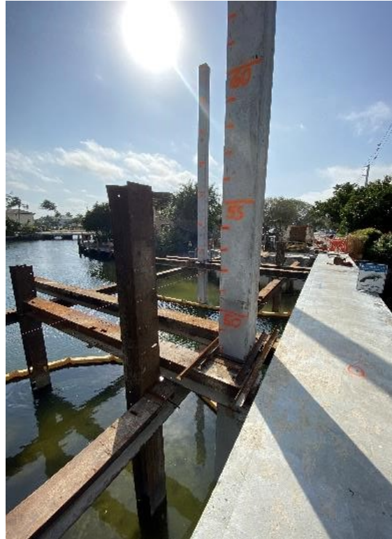
Pile installation challenging due to power lines and tight site conditions
