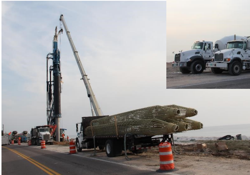
Secant-pile cages delivered to pile-drilling area and ready for installation
