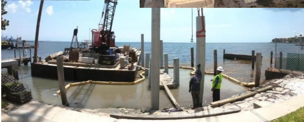
GFRP Cage Assembly, Casting and Installation of RC Piles
