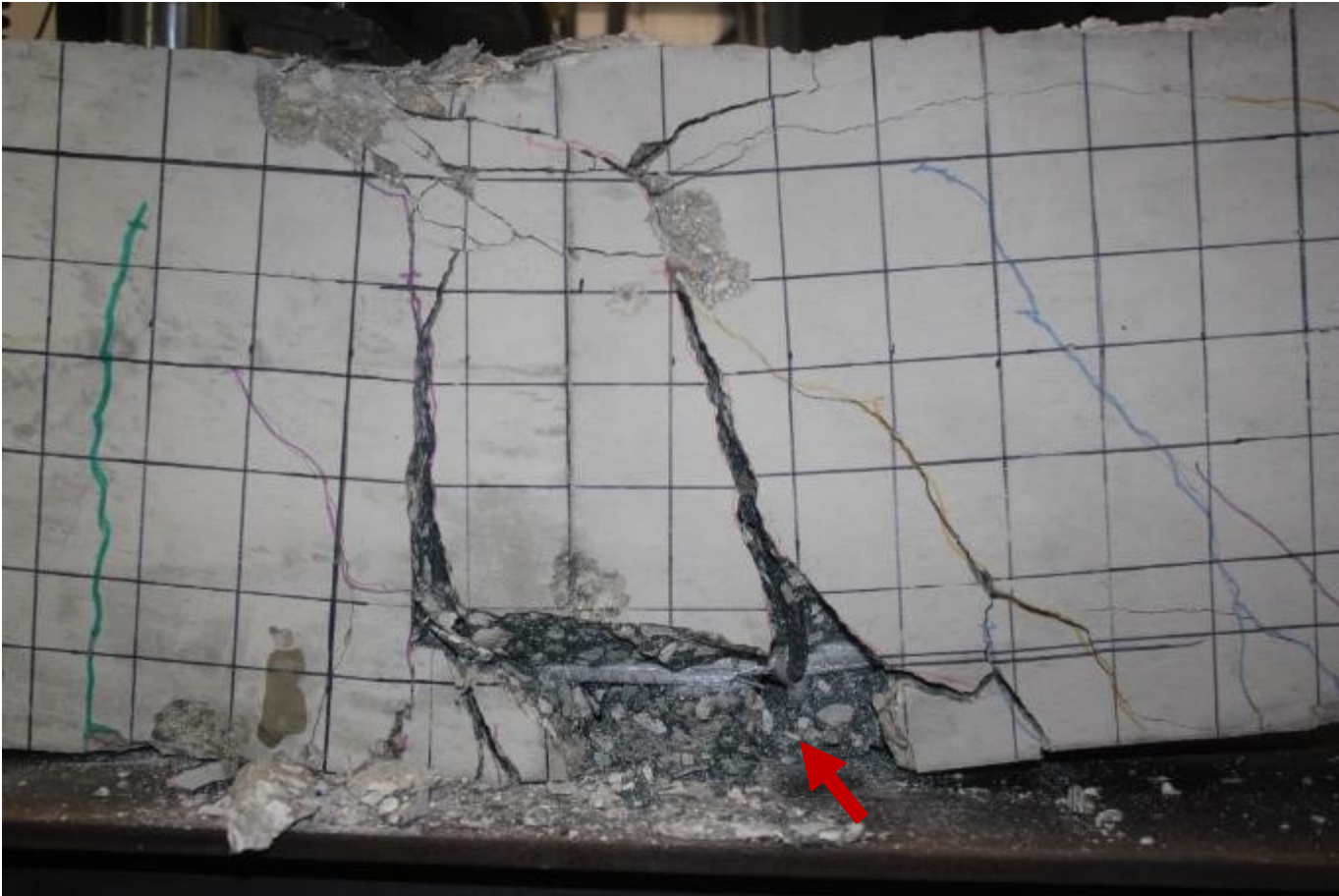
FRP Rupture Failure in GFRP Reinforced Beam
