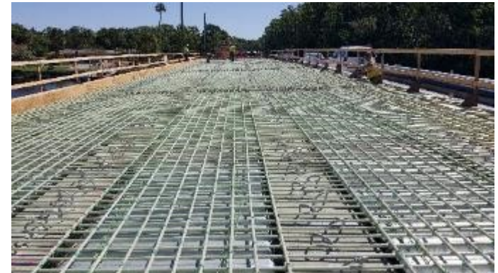
Deck of the Halls River Bridge in Homosassa (FL)
