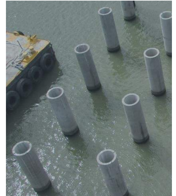
Precast concrete marine piles
