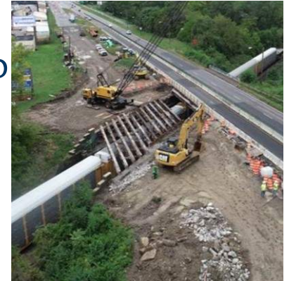
Anthony Wayne Trail Bridge
