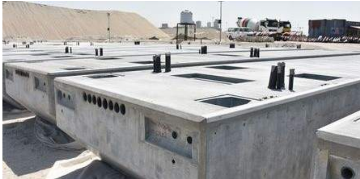
Precast concrete pontoons
