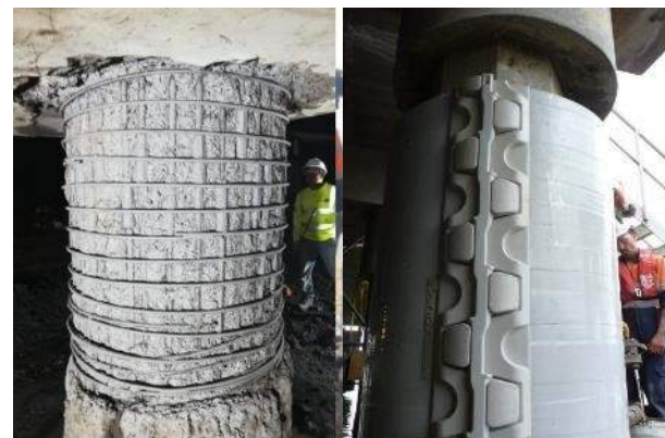
Rehabilitation of marine infrastructure
