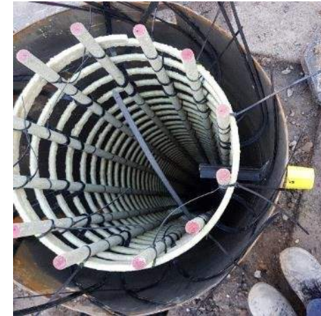
Pile cage in bored pier hole
