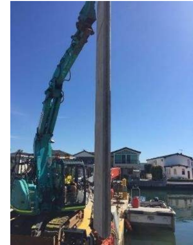
Seawall replacement, Sylvania Waters Sydney
