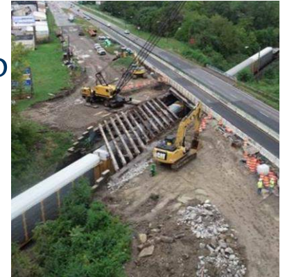
Anthony Wayne Trail Bridge
