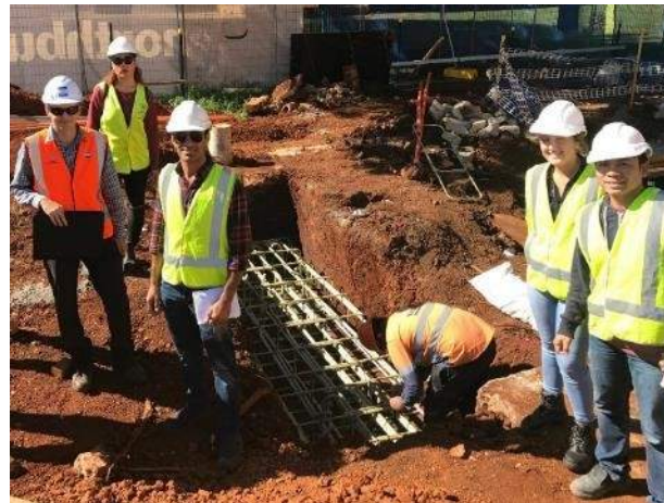
Annex extension, Toowoomba City Hall refurbishment project
