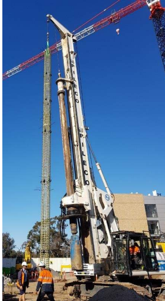
Lifting and installation of pile cage
