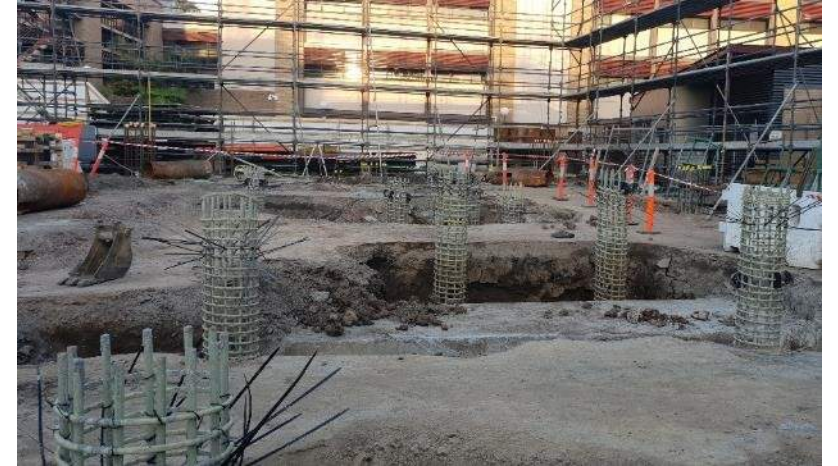
Pile cage in position
