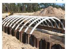
This project is the first installation of AIT Bridges' Composite Arch Bridge System in Florida. This project features our widest structure to date with an out to out width of 109 feet. The lower half of superstructure is submerged in final conditions. Fixed Fixed condition acheived with Carbon Fiber Composite Cable end cages installed at both ends of each arch.
