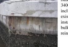
bulkhead cap on bridge 340003. Work activities included removal of the existing bulkhead cap and installation of a new bulkhead cap with GFRP reinforcement. Overall Budget/Cost Estimate: What was unique about this project?
