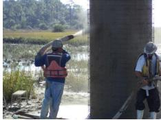
**Columns:** No. 4 L-shape GFRP dowel bars with epoxy were embedded into the columns to attach the 150mm x 150mm x
