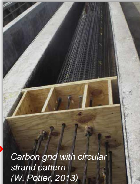
Prefabricated Auger-Cast-Pile FRP cages (Claura, et.al, 2015)
